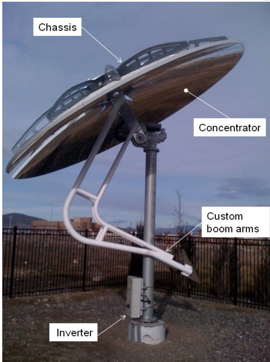
Figure 1, PowerDish™ Concentrator Modified for TES
