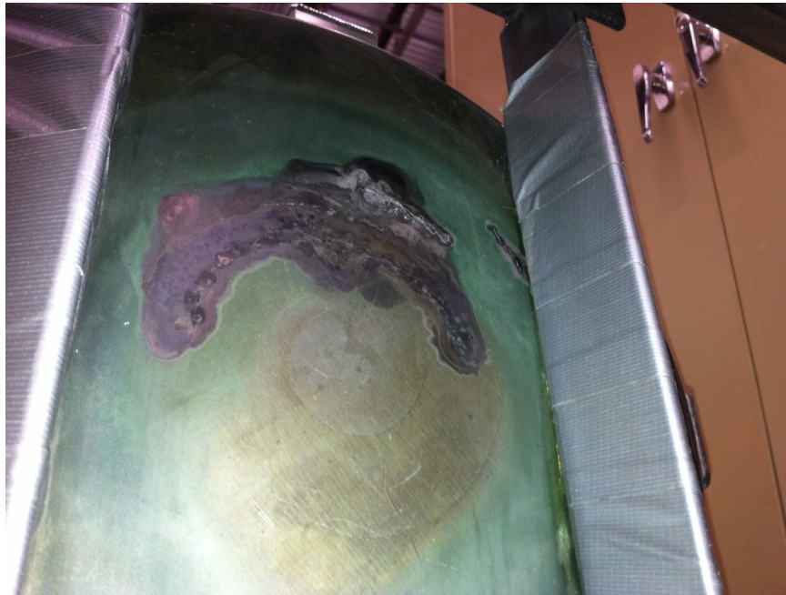
Figure 12, Test #1 Receiver Damage
