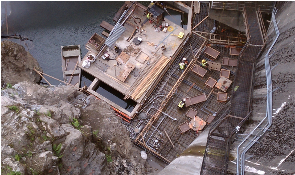
Preparation of powerhouse floor slab
