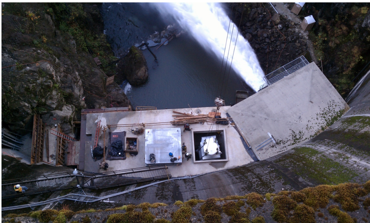
Lowering generators through roof and control floor
