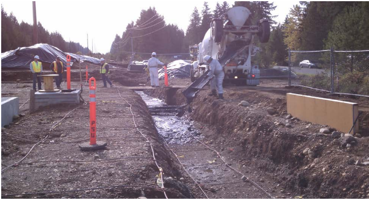
GEM slurry being poured into perimeter grounding trench
