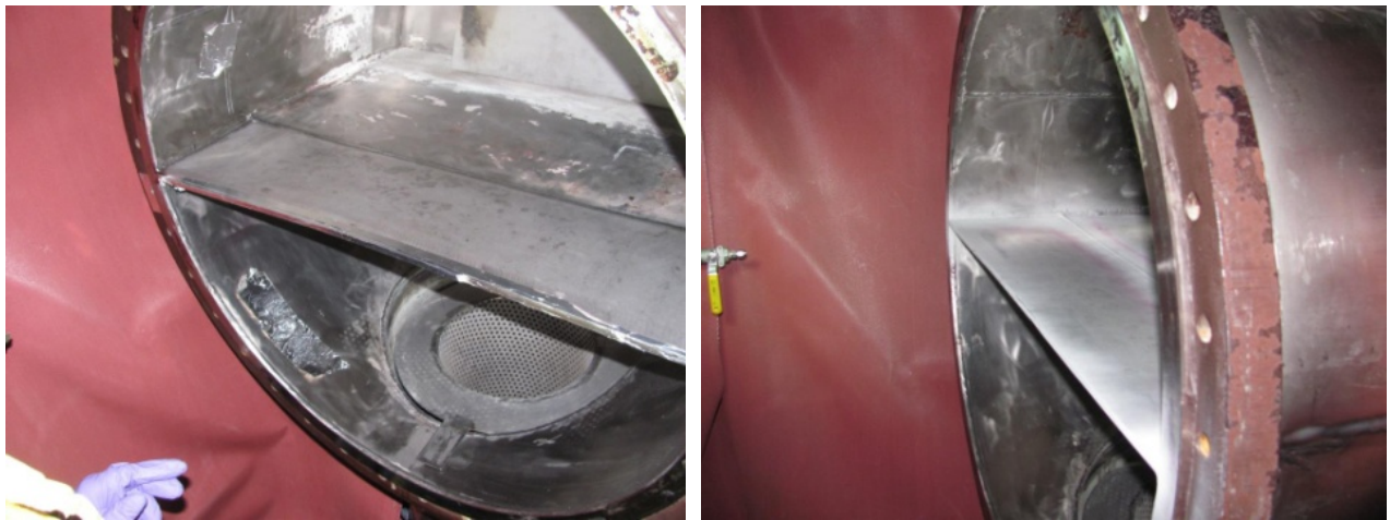
Figure 7. New piece of Inconel plate installed and inspected.
