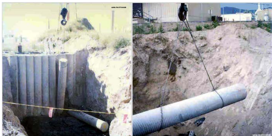
Figure 11. Removal of CMP from the Vertical Array
