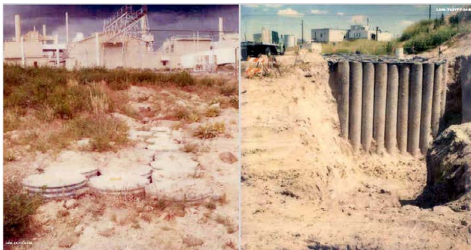
Figure 9. CMPs at Start of Retrieval from MDA T in 1986
