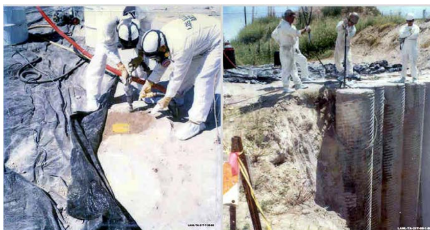
Figure 10. Preparation of CMPs for Removal from Vertical Array
