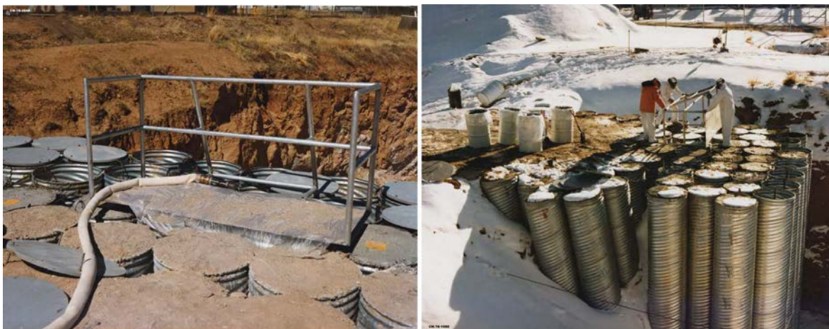
Figure 8. Filling CMPs with Retrievable Cement Paste (1978)
