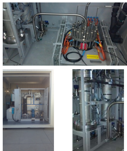
Figure 20. Electrolyzer Stack (top), Oxygen Chamber (bottom left), and Hydrogen Dryer (bottom right)
