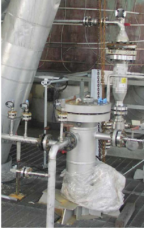
Photo 3.1.1 - Cyclone Vessel (left) and Gas Filtration Unit (right) as installed at the Wabash site
