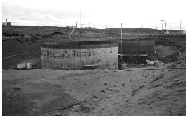
Figure 4-12. Vertical Concrete Shell Pouring (56710-9 Photo) (12/21/71)
