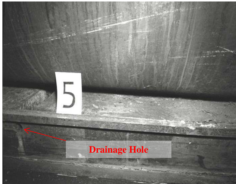
Figure 5-4. Kaolite Retaining Ring with 1 in. Drainage Hole Drilled at Air Channel
