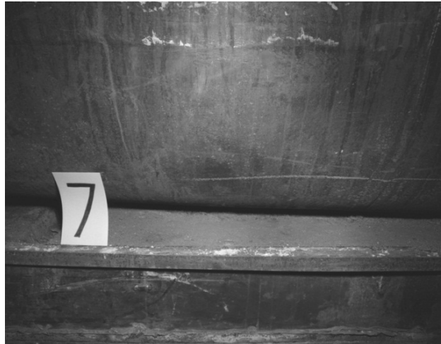
Figure 5-6. Kaolite Condition (Damp, Soft for 1/8 in. Depth) (57482-18 Photo) (Taken 3/24/72)
