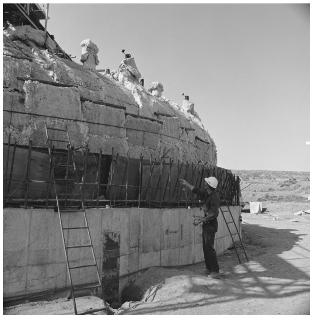
Figure 4-18. Insulation Installed and Held in Place with Wire Mesh on Tank AZ-102. (58073-4 Photo) (Taken 5/25/72)
