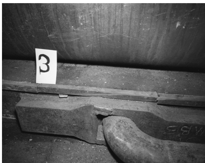
Figure 5-3. 2 in. Bar Welded to the Retainer Ring to Support Air Distribution Piping (57482-17 Photo) (Taken 3/24/72)
