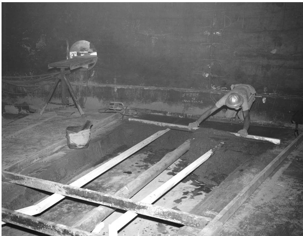
Figure 4-9. Tank AZ-101 Forms Placed and Refractory Being Poured (55952-6 Photo) (Taken 9/17/71)
