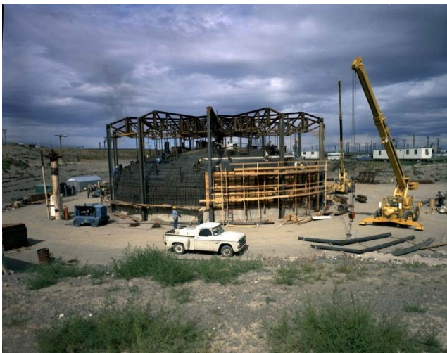
Figure 4-23. Tank AZ-101 Reinforcing Steel and Concrete Forms Being Placed on Tank AZ-101 (58324-2cn Photo) (Taken 6/23/72)
