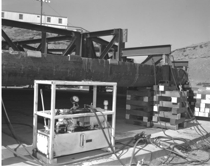
Figure 4-5. Secondary Liner Raised with Cribbing and Superstructure (55808-4 Photo) (Taken 8/30/71)
