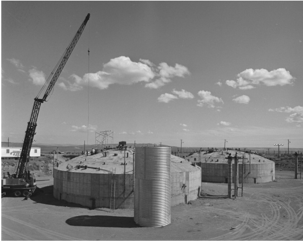
Figure 4-25. Overall View of 241-AZ Tank Farm Following Concrete Dome Completion (58744-40 Photo) (Taken 8/22/72)
