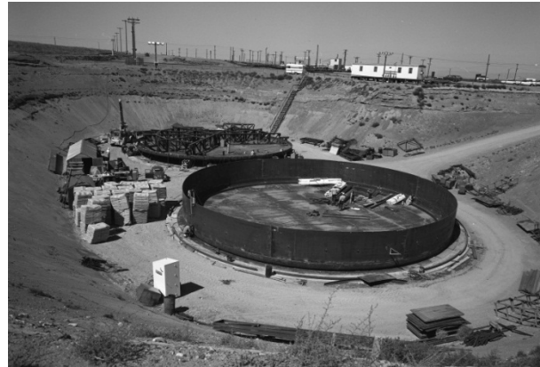
Figure 4-3. Viewing Erection of the Two Tanks' Secondary Liners (55748-6 Photo) (Taken 8/25/71)
