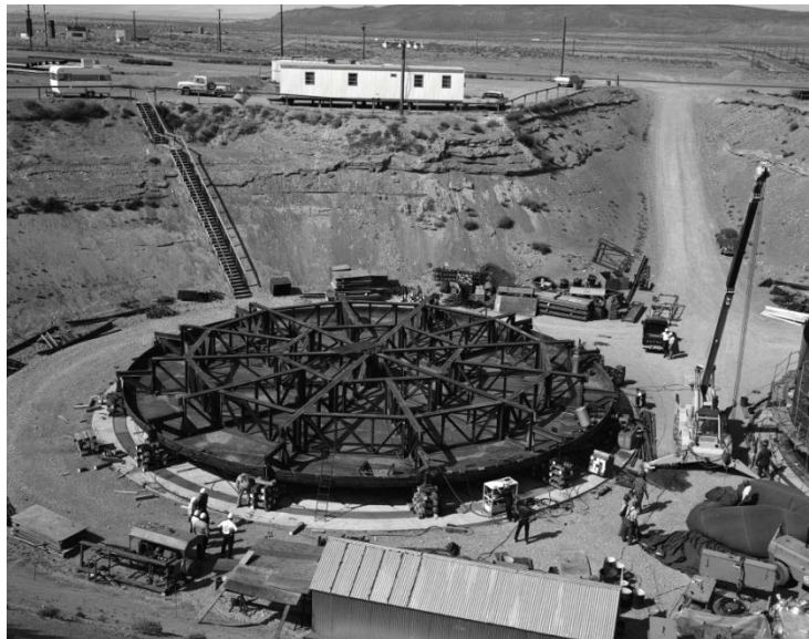
Figure 4-4. Constructing Secondary Liner – Looking North (55808-3 Photo) (Taken 8/30/71)
