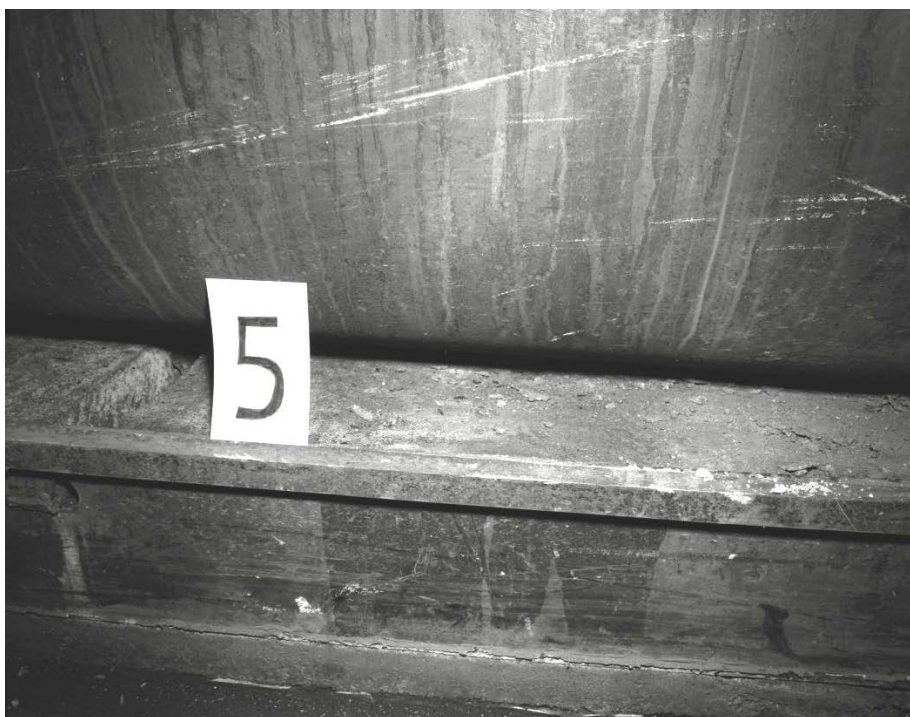
Figure 5-8. Kaolite Condition (1/8 in. Crust) (57482-19 Photo) (Taken 3/24/72)
