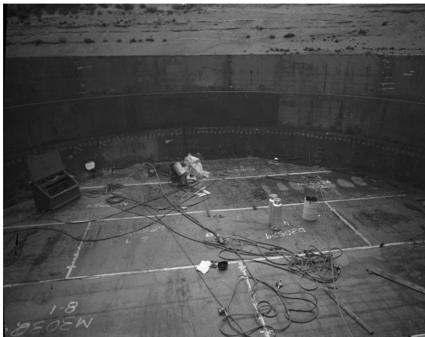
Figure 4-15 Weld Repairs in Progress on Tank AZ-102 – Looking South (56272-4 Photo) (Taken 10/26/71)
