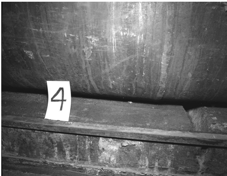
Figure 5-7. Kaolite Condition (Soggy and Mushy for 1/8 in. Depth) (57482-21 Photo) (Taken 3/24/72)
