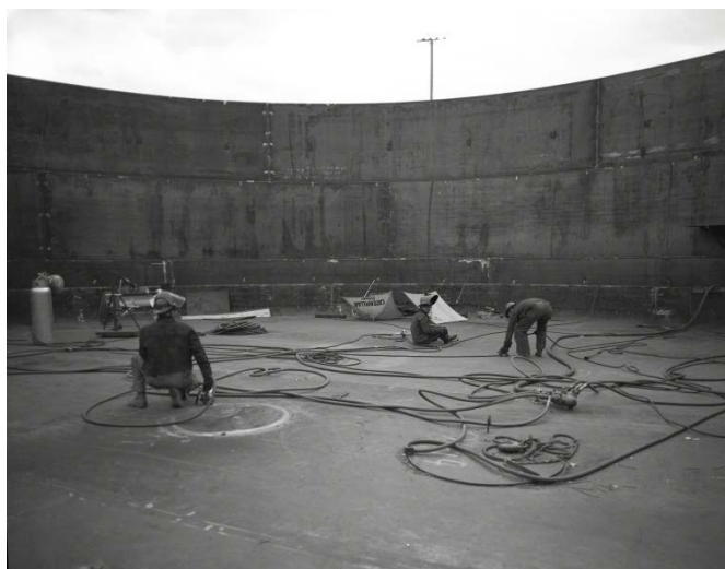
Figure 4-14. Welders Repairing Welds on the Primary Tank Bottom Sections Looking South, Tank AZ-101 (56272-6 Photo) (Taken 10/26/71)
