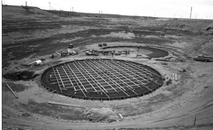
Figure 4-1. Progress on Tank Bases – Looking West (54511-15 Photo) (Taken 3/22/71)
