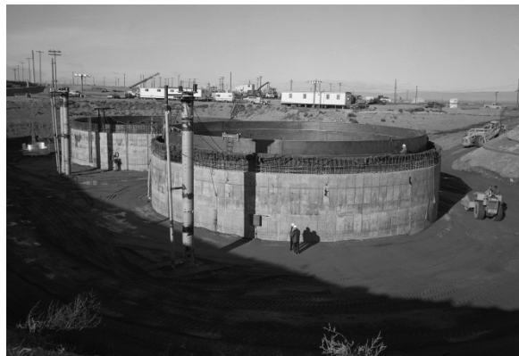
Figure 4-13. Backfilling Operations (56929-11 Photo) (Taken 1/21/72)
