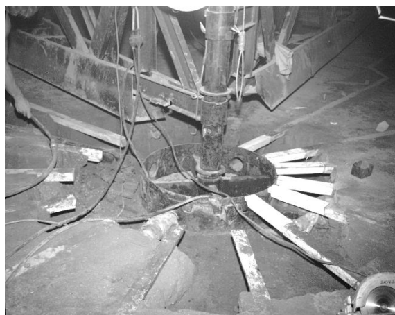
Figure 4-7. Tank AZ-101 Air Distribution Ring, 4 in. Air Supply Line, and Air Distribution Channels (55952-3 Photo) (Taken 9/17/71)
