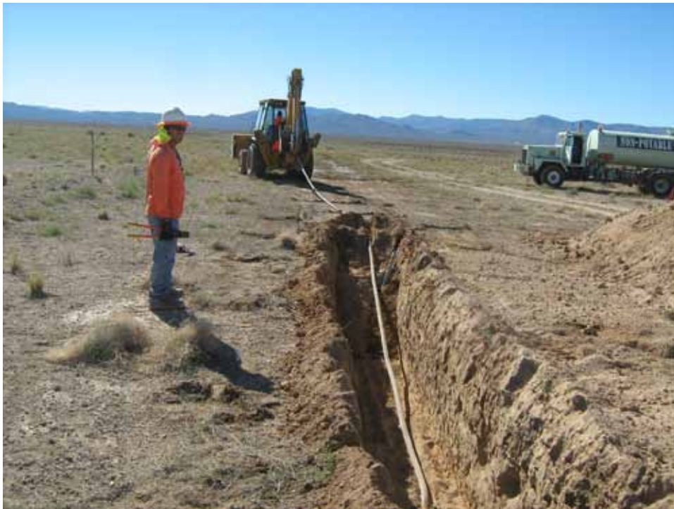
Photograph 4: Removal of Lead-Sheathed Cable, 10/30/2012
