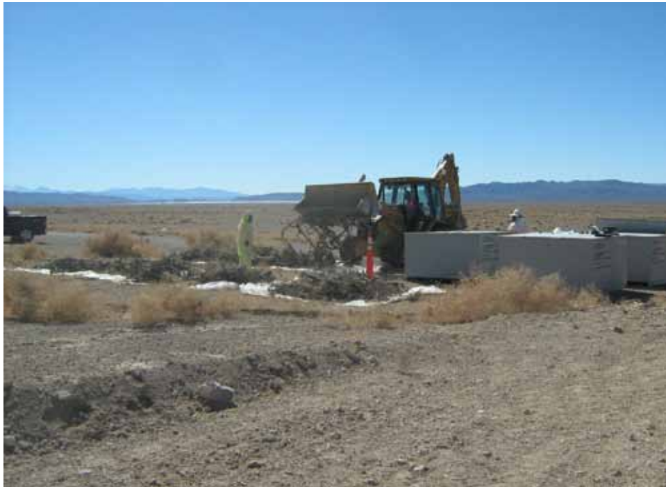
Photograph 20: Packaging Lead-Sheathed Cable Debris from the Berms into Macroencapsulation Boxes, 02/05/2013
