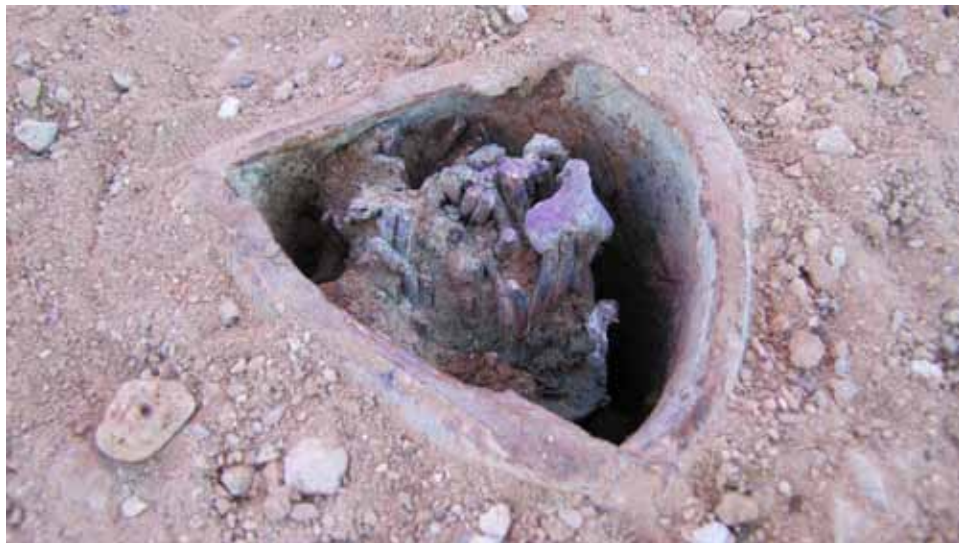
Photograph 18: Lead-Sheathed Cable and Steel Conduit at the Surface of the Concrete Pad, 01/30/2013
