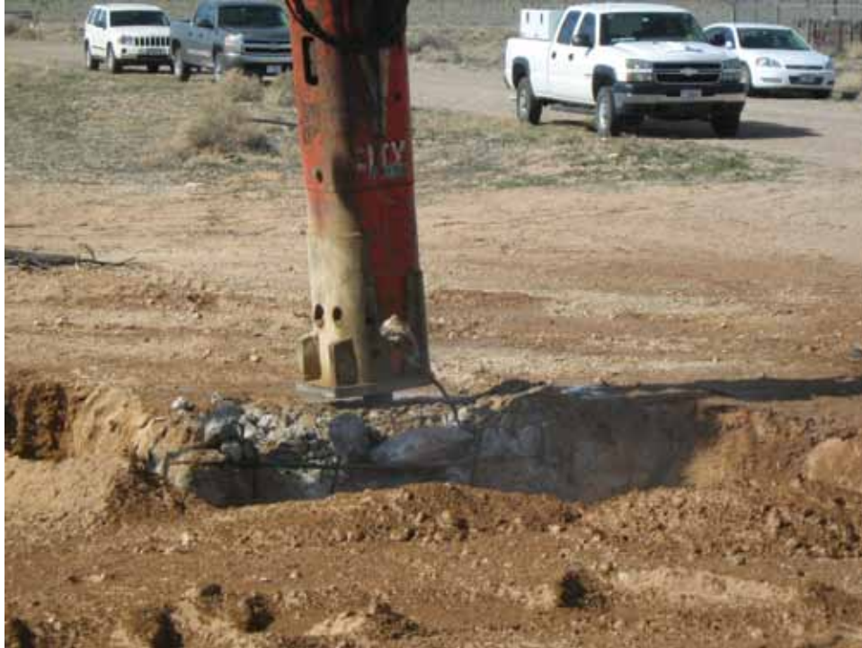
Photograph 26: Demolition of the Concrete Pad Where the Lead-Sheathed Cable Ended, 03/14/2013
