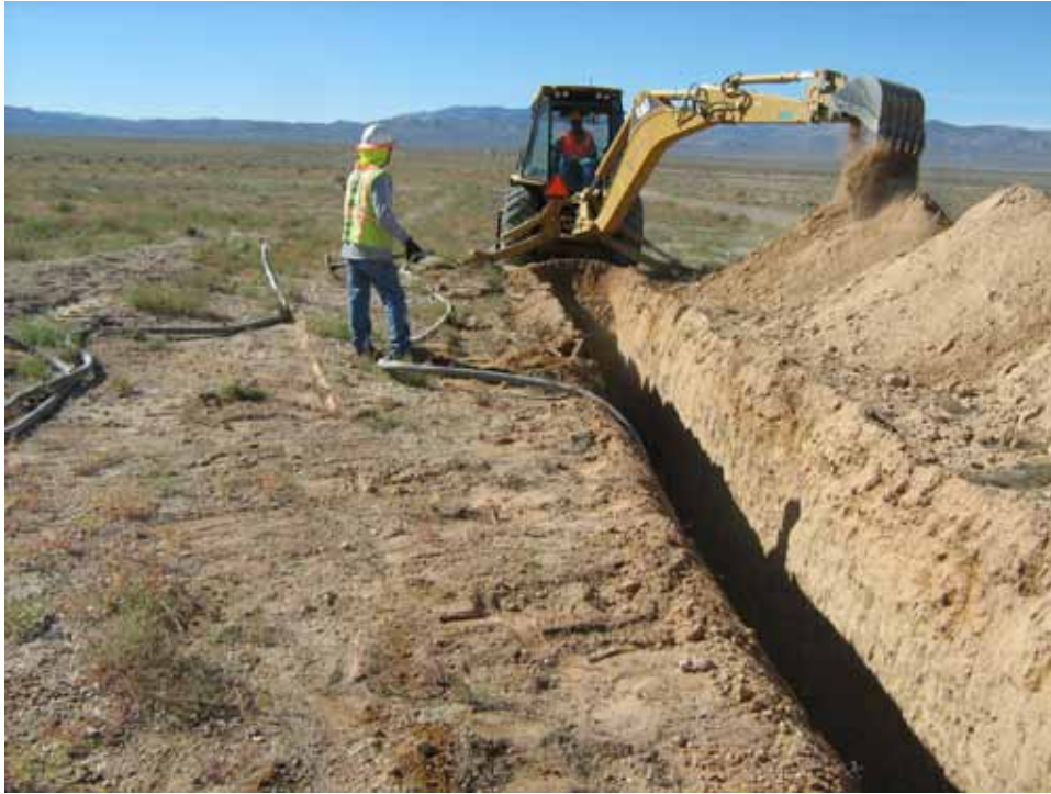
Photograph 5: Removal of Lead-Sheathed Cable, 10/31/2012
