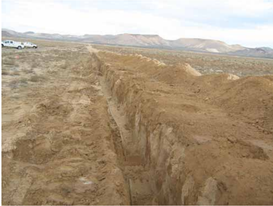
Photograph 9: Removal of Lead-Sheathed Cable, 11/15/2012
