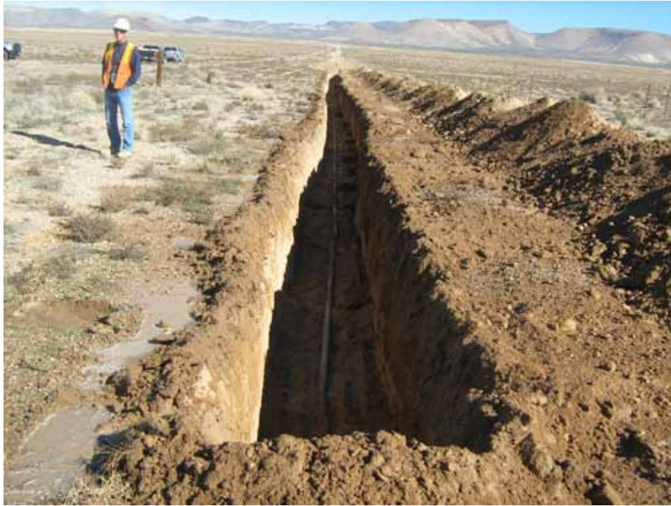
Photograph 11: Removal of Lead-Sheathed Cable, 11/20/2012
