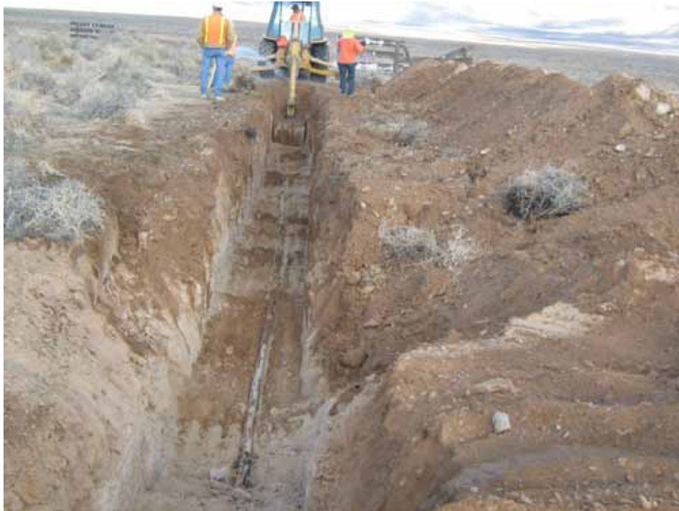
Photograph 15: Removal of Lead-Sheathed Cable, 12/03/2012
