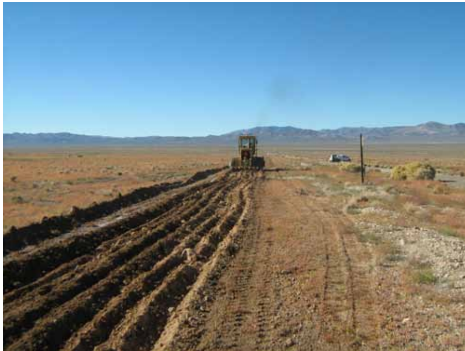
Photograph 8: Ripping the Berms, 11/07/2012
