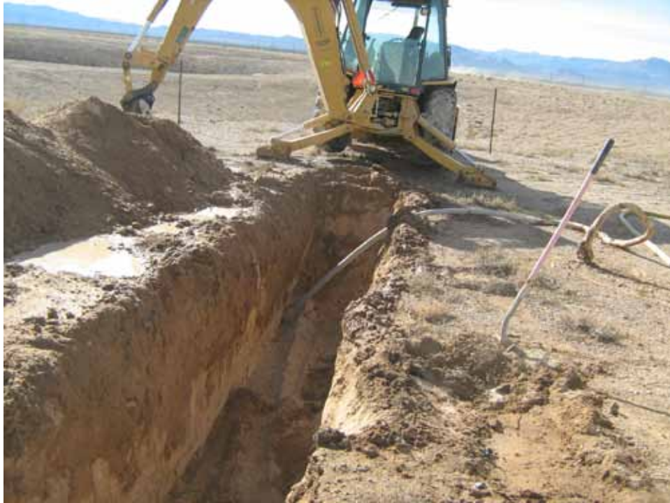
Photograph 13: Removal of Lead-Sheathed Cable, 11/28/2012
