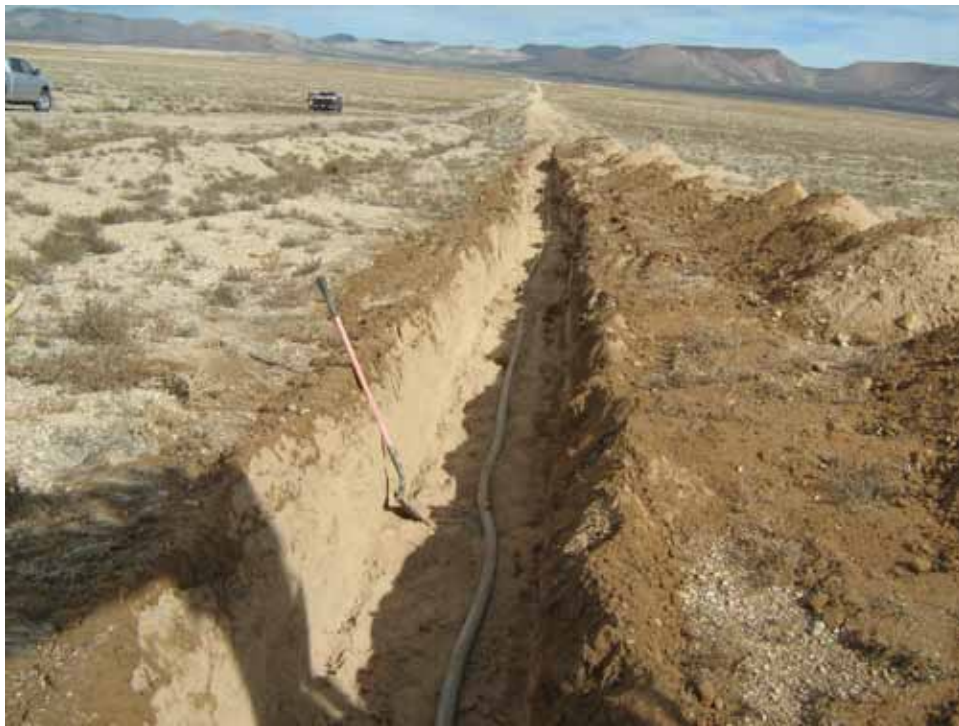
Photograph 12: Removal of Lead-Sheathed Cable, 11/21/2012
