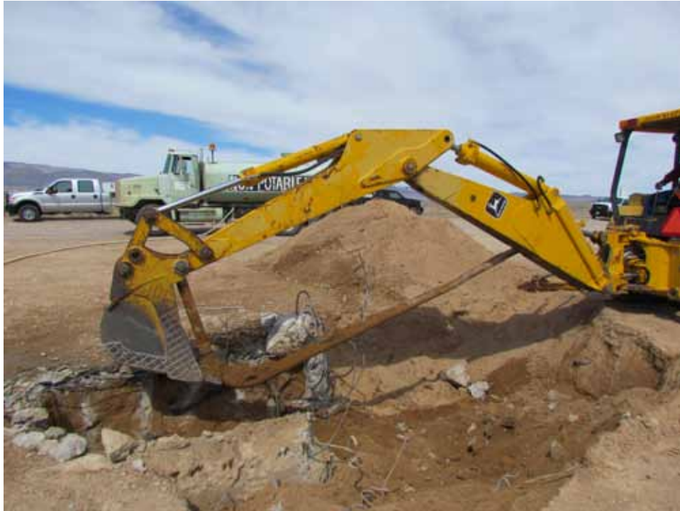
Photograph 27: Removal of the Steel Conduit and Lead-Sheathed Cable from the Concrete Pad, 03/14/2013
