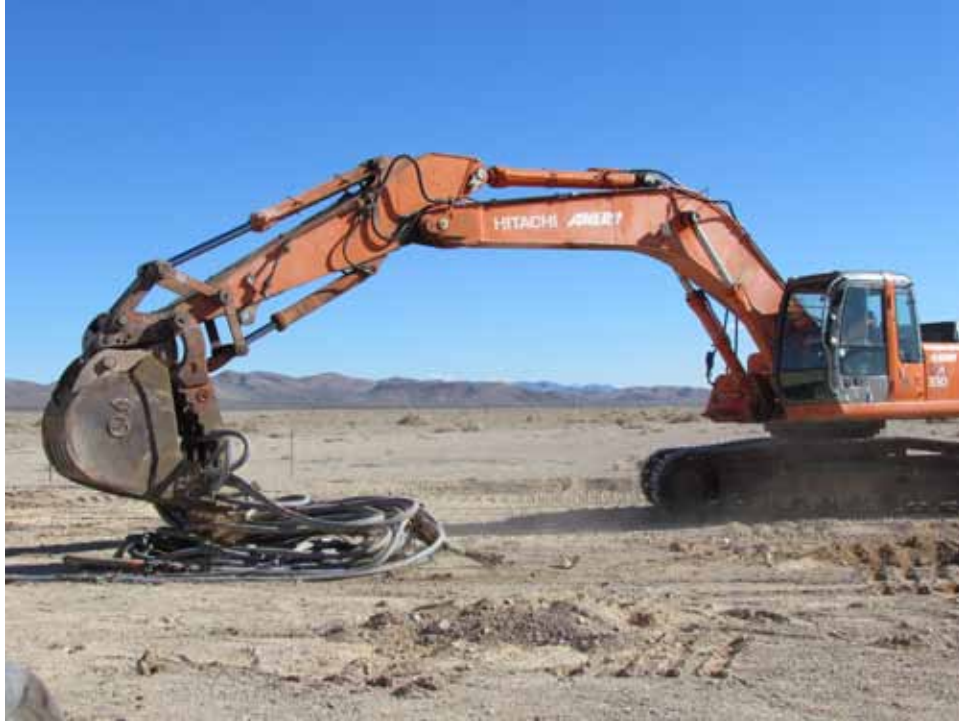
Photograph 23: Bundling the Long Sections of Lead-Sheathed Cable, 02/11/2013
