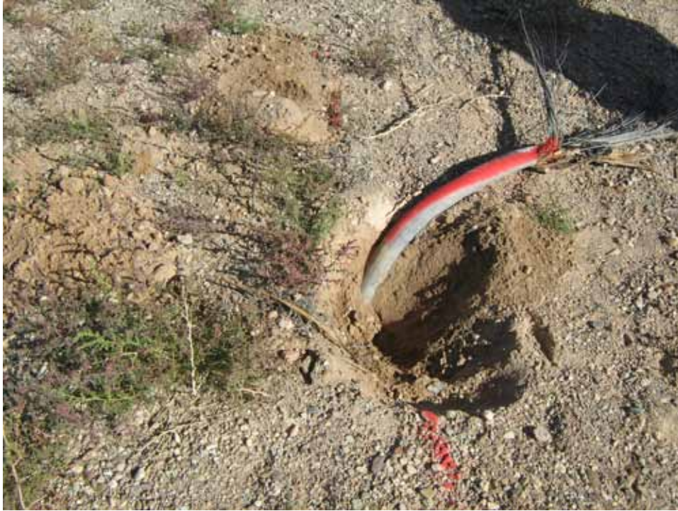
Photograph 1: Section of Lead-Sheathed Cable at Trench 4 Leading Underground, 10/23/2012
