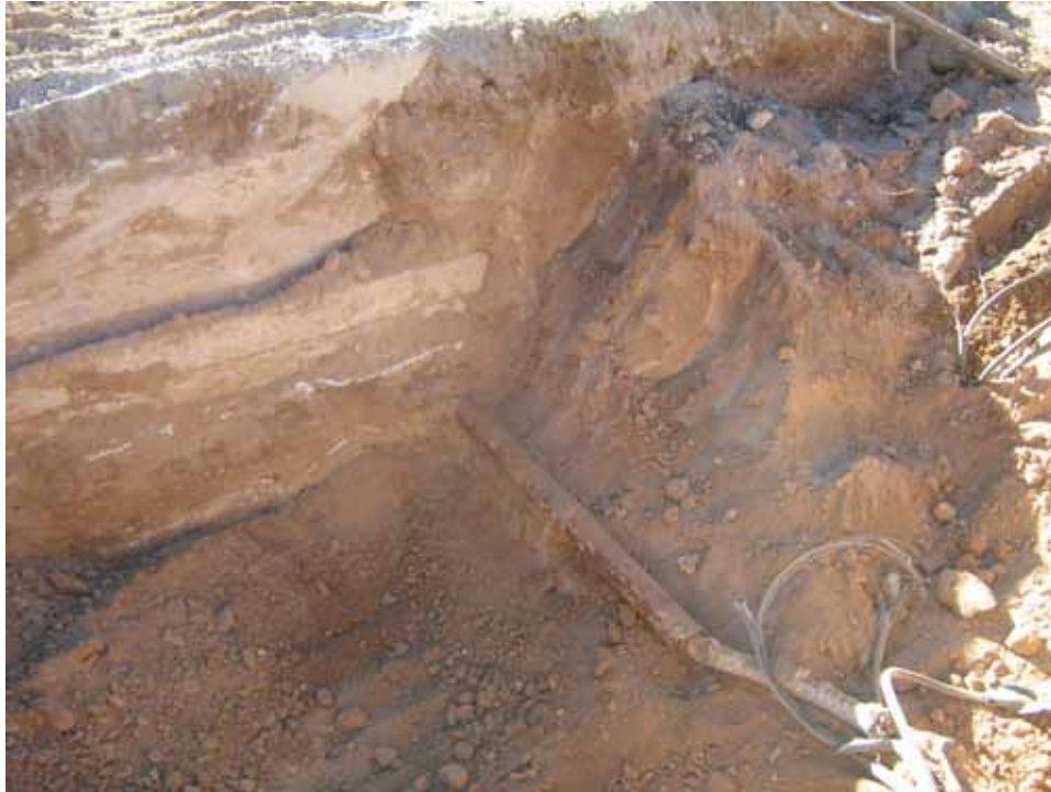
Photograph 17: Lead-Sheathed Cable and Steel Conduit under the Concrete Pad, 01/30/2013
