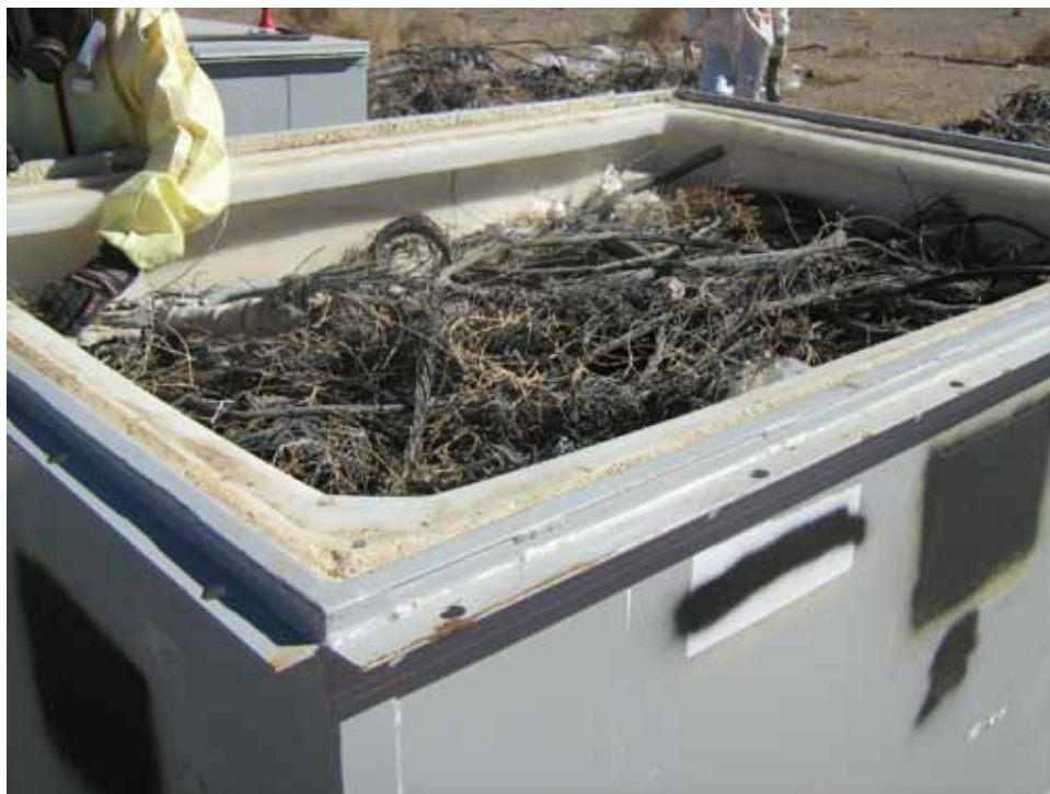
Photograph 21: Lead-Sheathed Cable Debris from the Berms in Macroencapsulation Box, 02/05/2013
