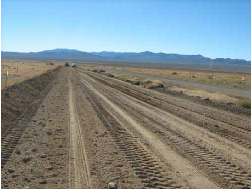
Photograph 7: Grading the Berms, 11/06/2012
