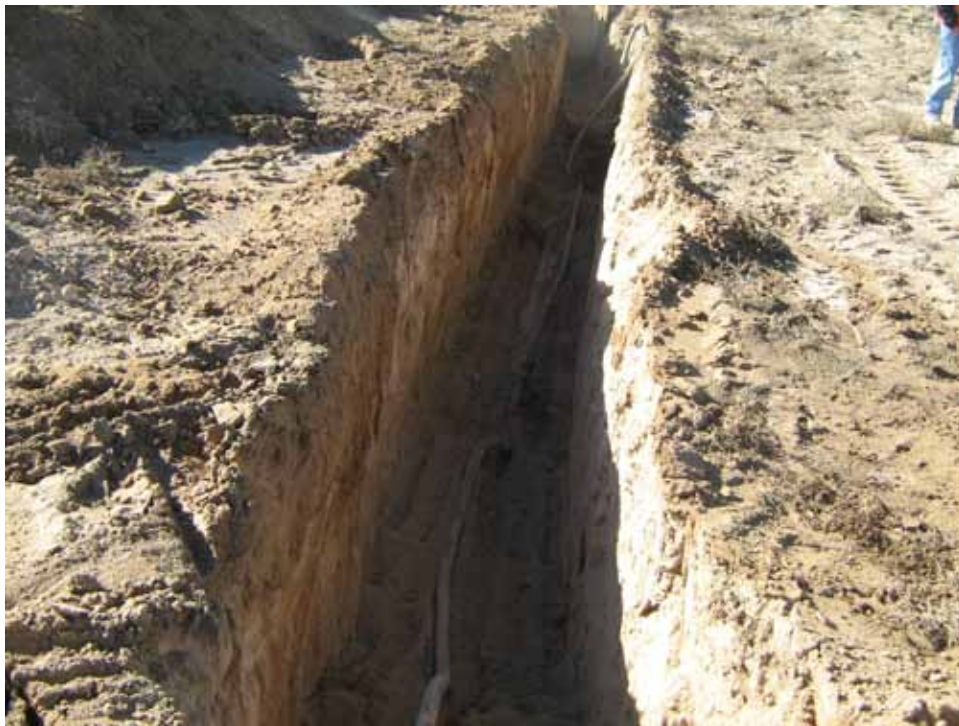
Photograph 10: Removal of Lead-Sheathed Cable, 11/19/2012
