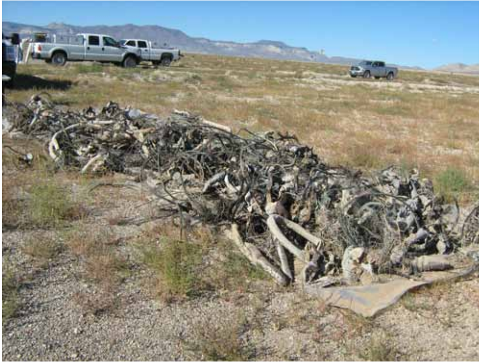
Photograph 3: Lead-Sheathed Cable Debris from Berm Staged on Plastic, 10/25/2012
