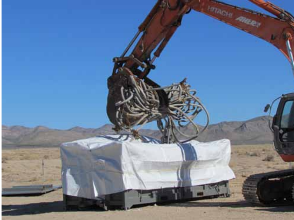
Photograph 24: Packaging the Long Sections of Lead-Sheathed Cable into an Intermodal Container, 02/11/2013
