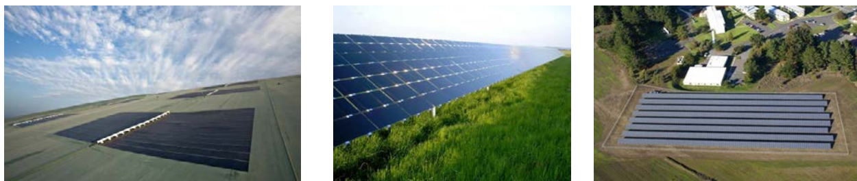
Figure 4. Thin-film solar panels installed on (left) landfill geomembrane cover and (middle/right) fixed-tilt mounting system. Photos from (left) Republic Services, Inc., NREL 23817; (middle) Beck Energy, NREL 14726; and (right) U.S. Coast Guard Petaluma site, NREL 17395
