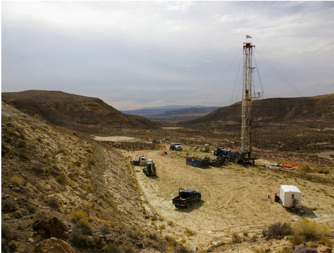
Figure 18. A picture taken when the monitoring geophone string was cemented into well C313SE in October, 2007 for microseismic and time-lapse offset VSP monitoring.
