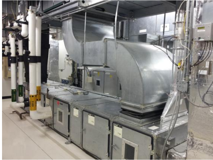
Figure 11. Test System Air Handling Unit
