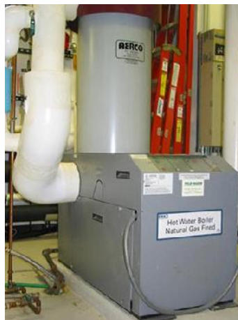
Figure 16. Natural Gas-Fired Boiler
