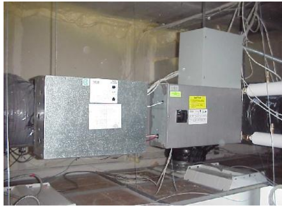
Figure 13. Variable-Air-Volume Terminal Unit
