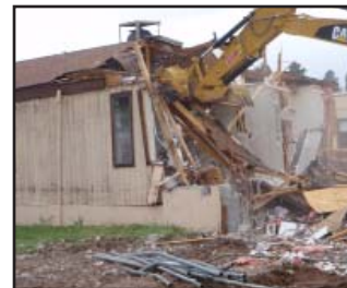
D&D of Temporary Structures
