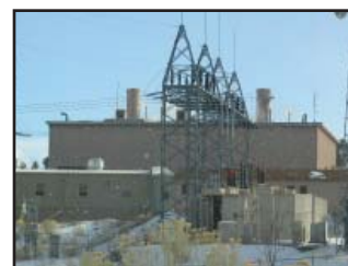
Replacement of the TA-3 Steam Plant
