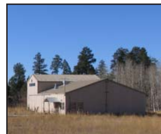
Aging/Obsolete Facility at Fenton Hill
