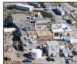
Radioactive Liquid Waste Treatment Facility (RLWTF) Upgrades
