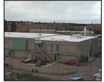
Beryllium Technology Facility (BTF)
