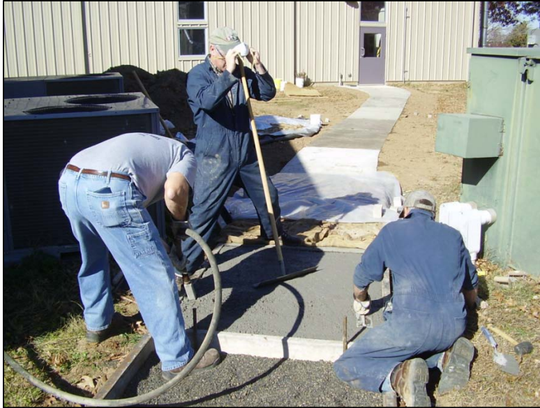
Figure 59. Placing and compacting a section of concrete.
