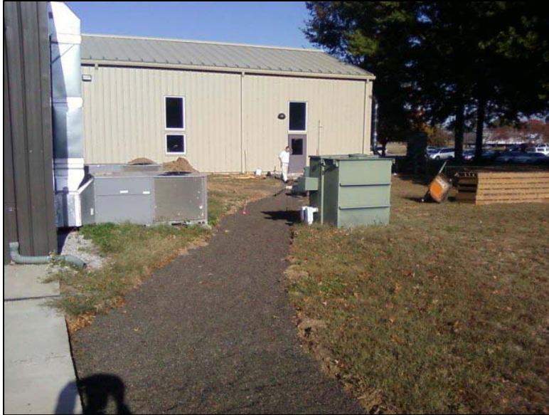
Figure 57. Walkway location showing bottom ash base course.
