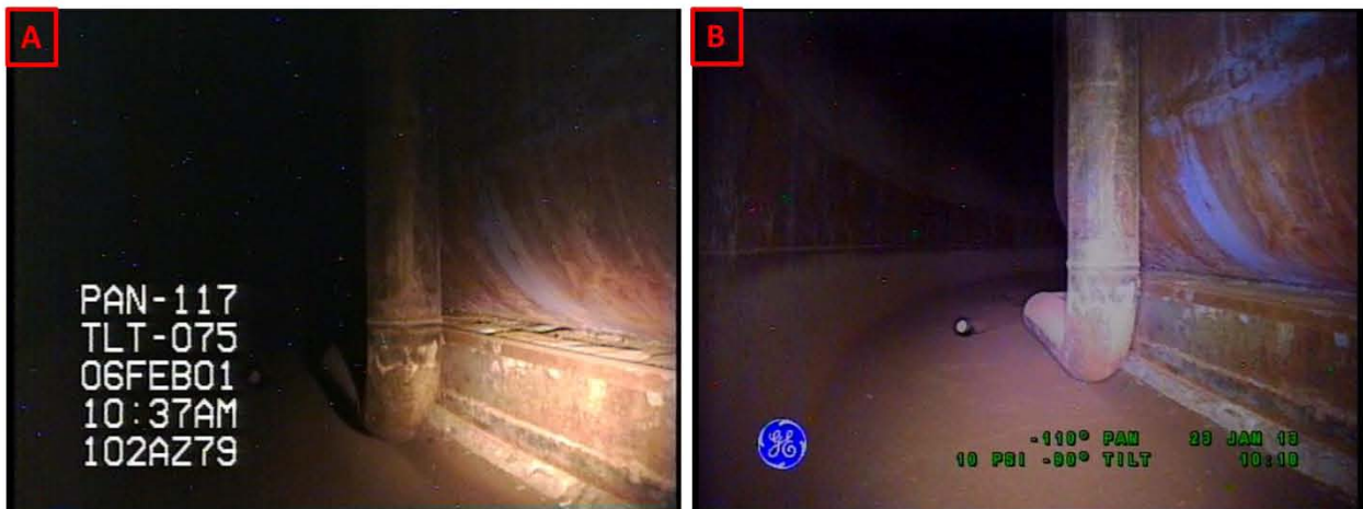
Figure 3-7. Riser 79 Lower Knuckle and Annulus Floor Comparisons Between Inspections on February 6, 2001 (A) and January 23, 2013 (B) Looking Towards Riser 80
