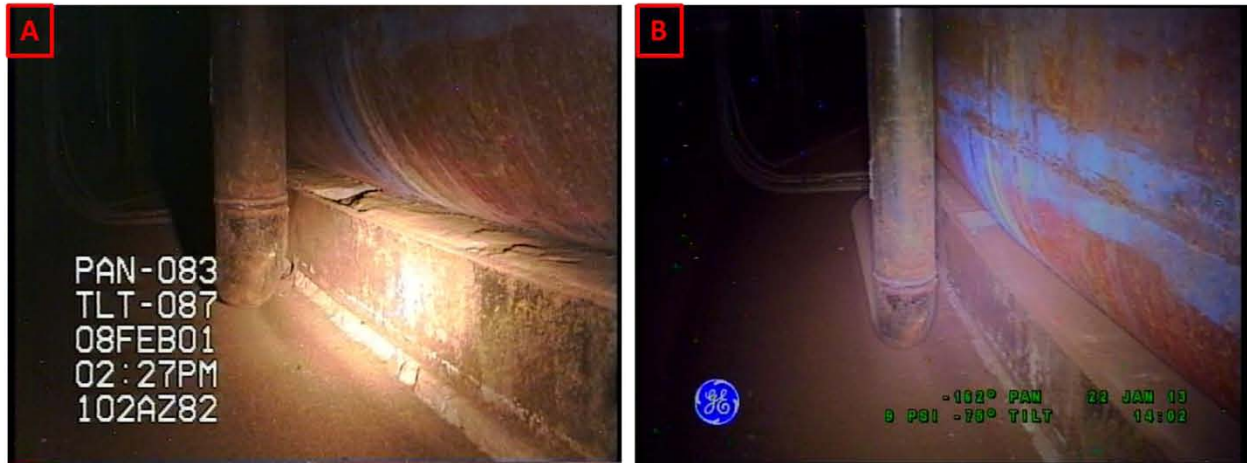
Figure 3-19. Riser 82 Lower Knuckle and Annulus Floor Comparisons Between Inspections on February 8, 2001 (A) and January 22, 2013 (B) Looking Towards Riser 95
