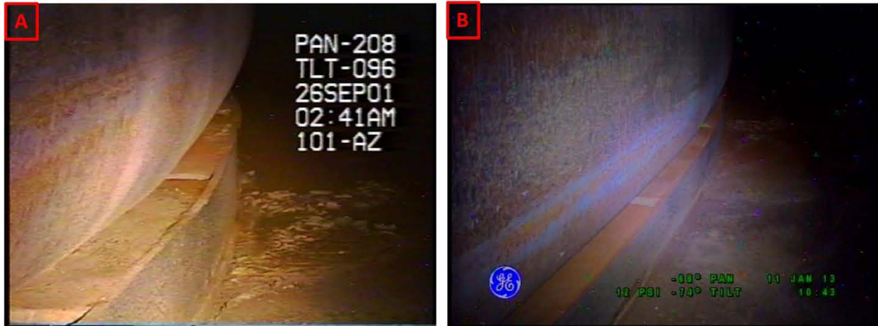
Figure 2-16. Riser 82 Lower Knuckle and Annulus Floor Comparisons Between Inspections on September 26, 2001 (A) and January 11, 2013 (B) Looking Towards Riser 105
