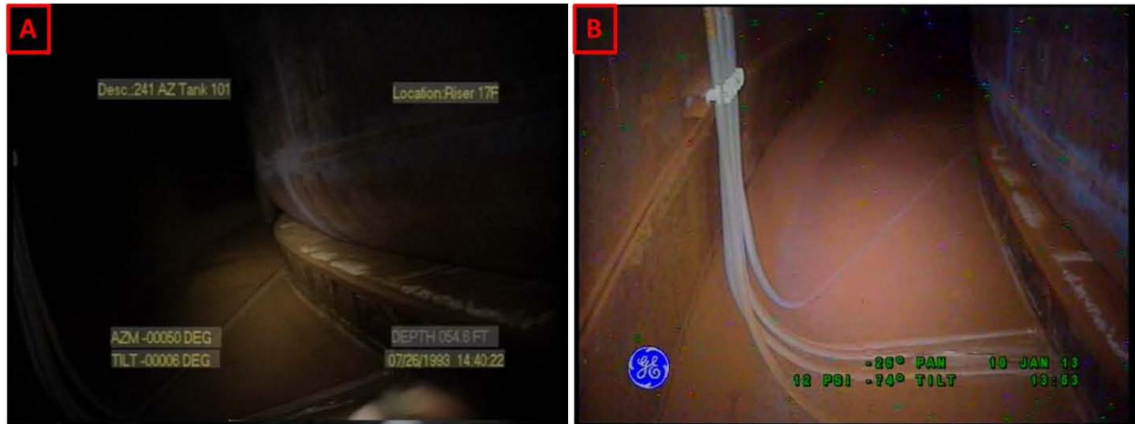
Figure 2-20. Riser 83 Lower Knuckle and Annulus Floor Comparisons Between Inspections on July 26, 1993 (A) and January 10, 2013 (B) Looking Towards Riser 96
