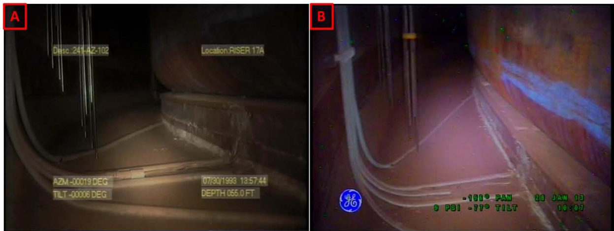
Figure 3-3. Riser 78 Lower Knuckle and Annulus Floor Comparisons Between Inspections on July 30, 1993 (A) and January 28, 2013 (B) Looking Towards Riser 93
