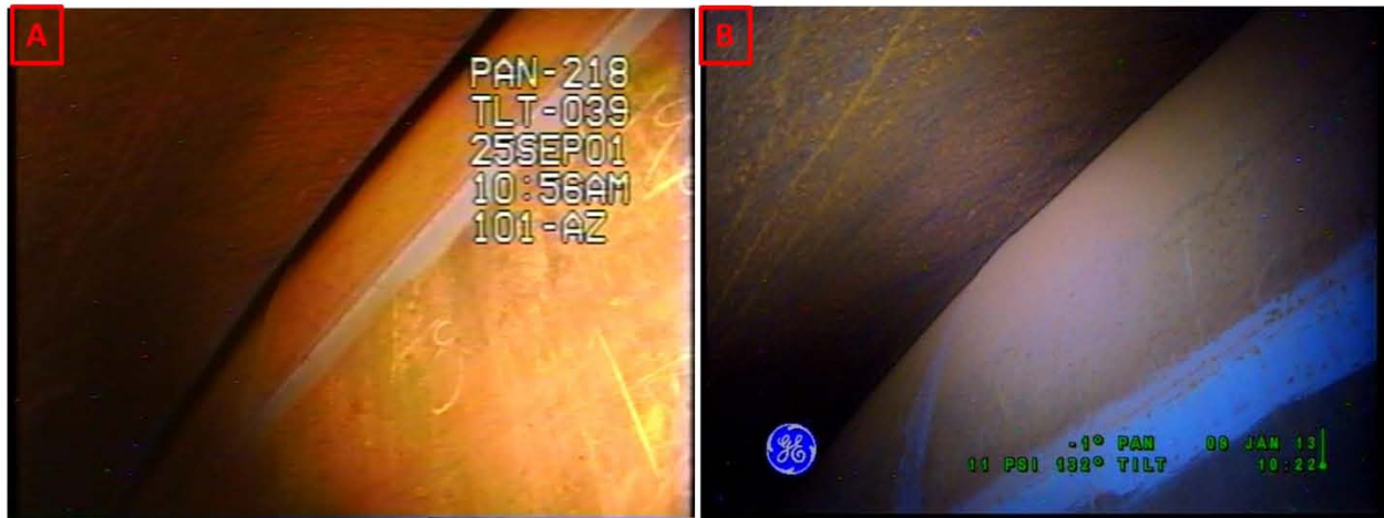
Figure 2-1. Riser 78 Upper Haunch Comparisons Between Inspections on September 25, 2001 (A) and January 9, 2013 (B) Looking Towards Riser 93
