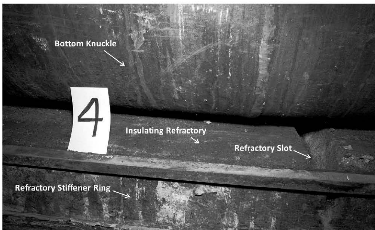
Figure 1-4. 241-AZ Farm Tank Annulus Description Showing Refractory Slot (N1641598)
