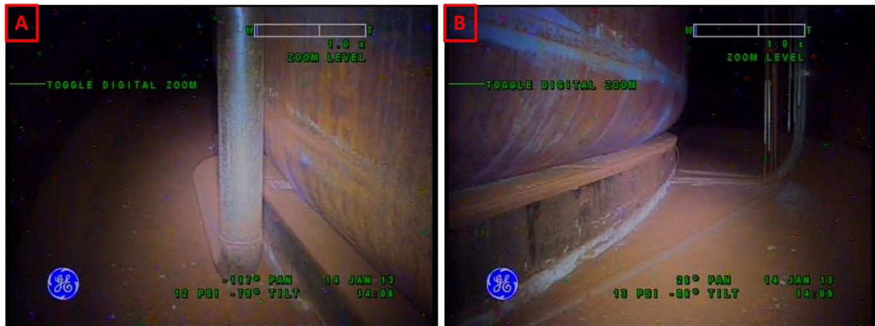
Figure 2-8. Riser 79 Lower Knuckle and Annulus Floor Condition on January 14, 2013 Looking Towards Riser 80 (A) and Looking Towards Riser 99 (B)
