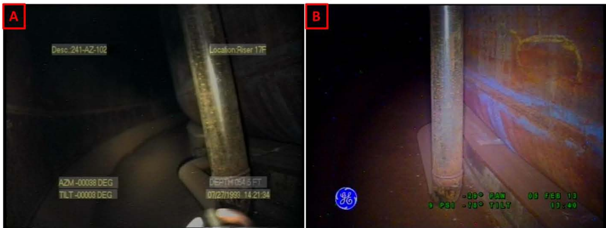
Figure 3-26. Riser 84 Lower Knuckle and Annulus Floor Comparisons Between Inspections on July 27, 1993 (A) and February 5, 2013 (B) Looking Towards Riser 85
