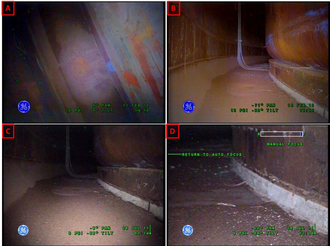
Figure 4-2. Annulus Floor Discoloration in Tank AZ-102 as seen from Riser 92 in 2013 (A), from Riser 80 in 2013 (B), from Riser 80 in 2011 (C), and Close Up View Showing Elevation Differences as seen from Riser 80 in 2011 (D)
