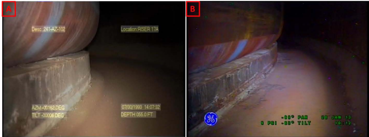
Figure 3-4. Riser 78 Lower Knuckle and Annulus Floor Comparisons Between Inspections on July 30, 1993 (A) and January 28, 2013 (B) Looking Towards Riser 90
