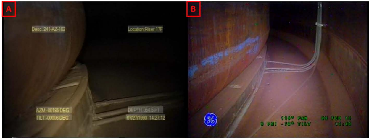
Figure 3-27. Riser 84 Lower Knuckle and Annulus Floor Comparisons Between Inspections on July 27, 1993 (A) and February 5, 2013 (B) Looking Towards Riser 102
