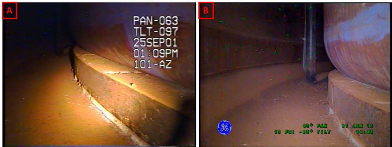
Figure 2-28. Riser 86 Lower Knuckle and Annulus Floor Comparisons Between Inspections on September 25, 2001 (A) and January 7, 2013 (B) Looking Towards Riser 87
