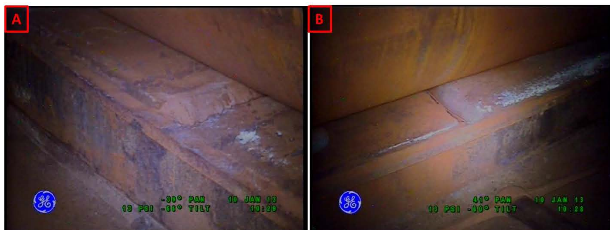
Figure 2-36. Riser 89 General Condition of the Refractory Slots on January 10, 2013
