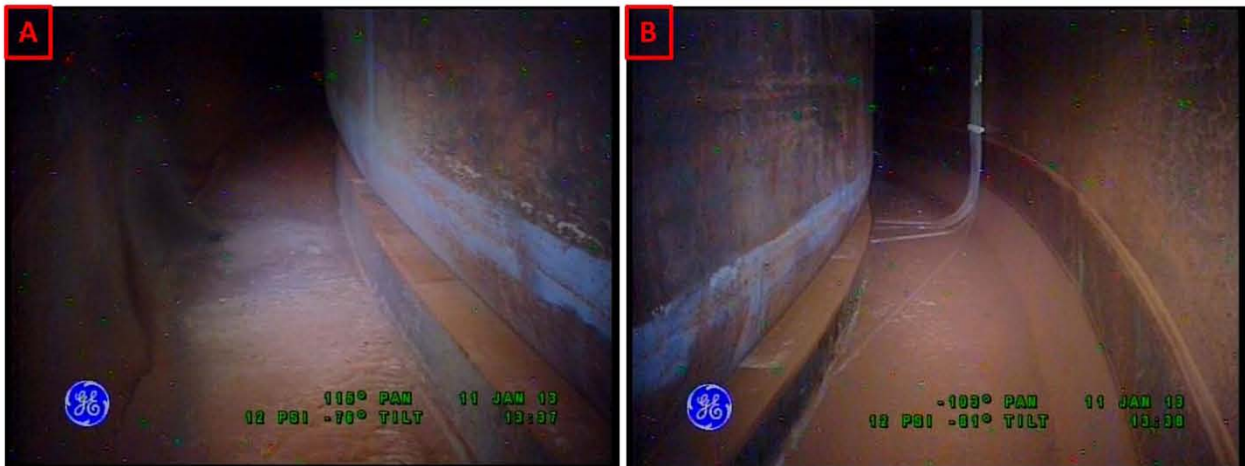
Figure 2-11. Riser 81 Lower Knuckle and Annulus Floor Condition on January 11, 2013 Looking Towards Riser 105 (A) and Looking Towards Riser 100 (B)
