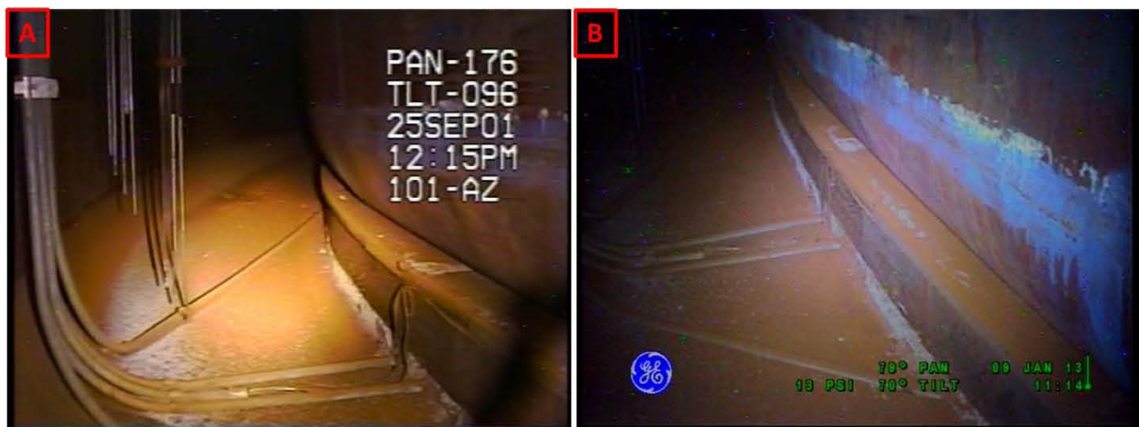
Figure 2-3. Riser 78 Lower Knuckle and Annulus Floor Comparisons Between Inspections on September 25, 2001 (A) and January 9, 2013 (B) Looking Towards Riser 93
