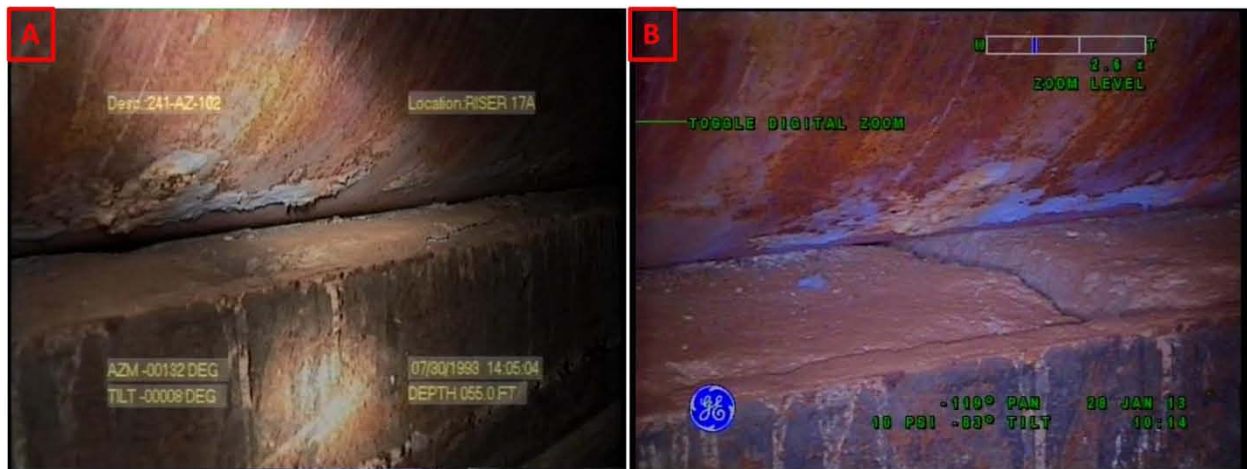
Figure 3-5. Riser 78 General Condition of the Refractory Slots on July 30, 1993 (A) and January 28, 2013 (B)
