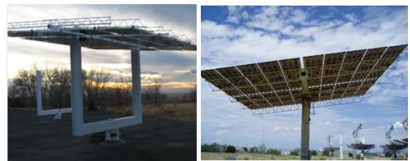
Figure 1: Representative heliostat designs. NSTTF heliostat (left) and ATS heliostat (right)
