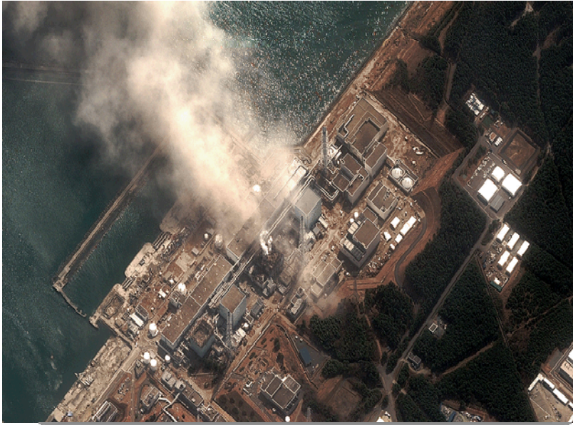
Fukushima Daiichi Nuclear Power Plant Accident
