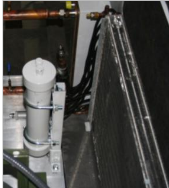
Figure 3-18: Accumulator and Evaporator with its Refrigerant Distributor
