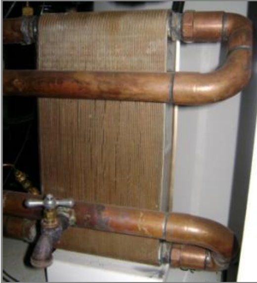
Figure 3-13: R134a Brazed Plate Condenser
