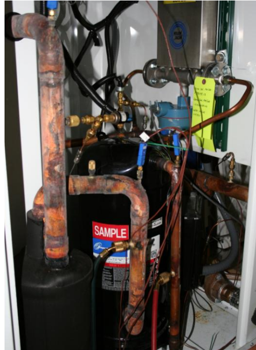
Figure 2-5: High Pressure Side of HPWH with Added Instrumentation
