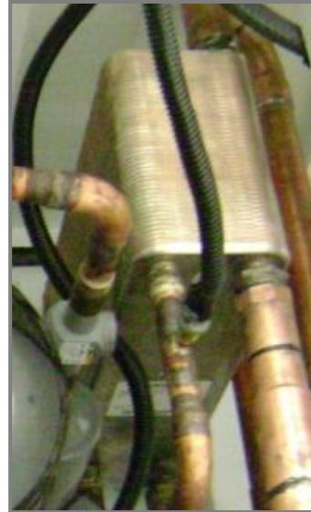
Figure 3-13: R134a Brazed Plate Condenser
