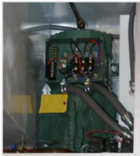
Figure 3-7: R744 Compressor in Heat Pump Housing
