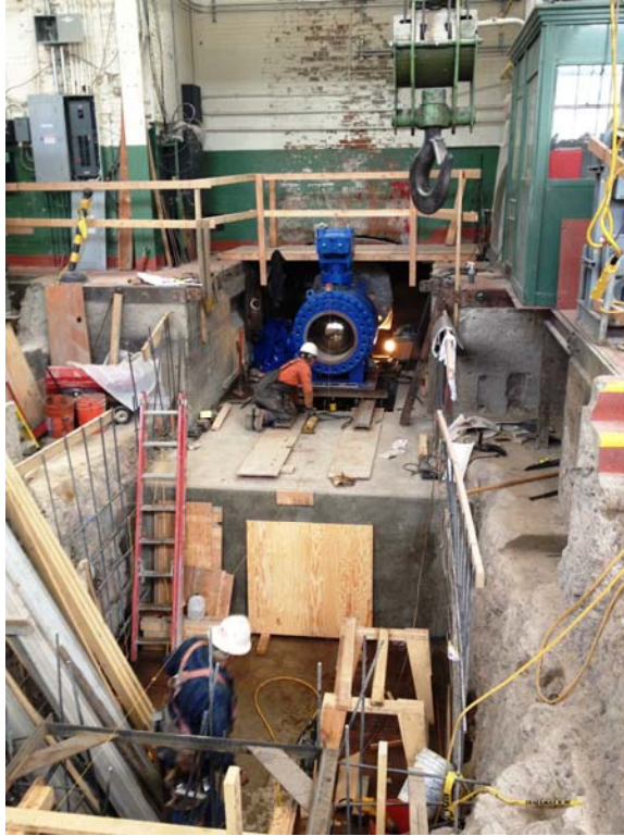
Figure 7 – Installation of New TIV (3/15/12)
