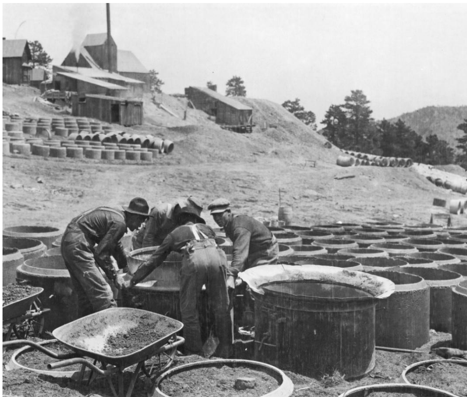
Figure 2. Workers fabricating steel-reinforced concrete gravity pipeline sections at one of the work sites (perhaps Magnolia work camp) established during the project.
