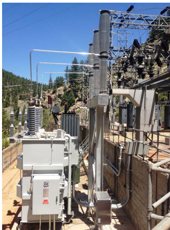
Figure 16 – Circuit Switcher Install (5/15/12)
