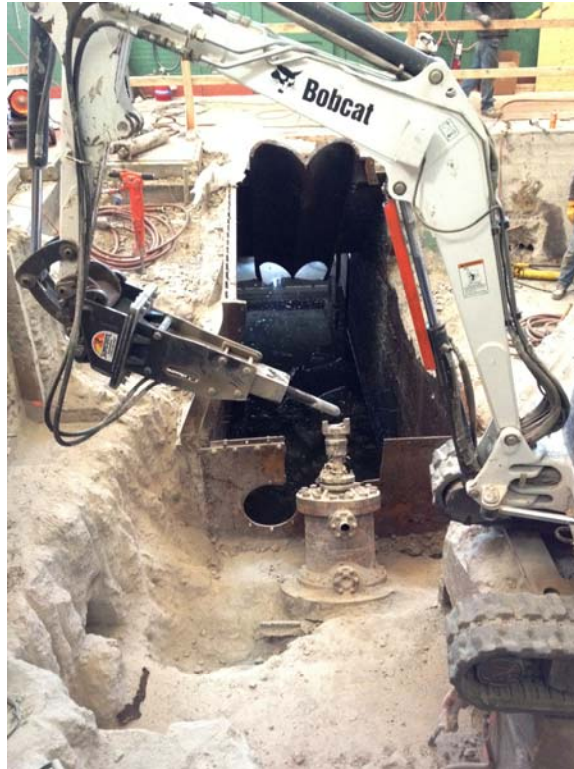
Figure 3 – Turbine Pit Concrete Demo (1/12/12)
