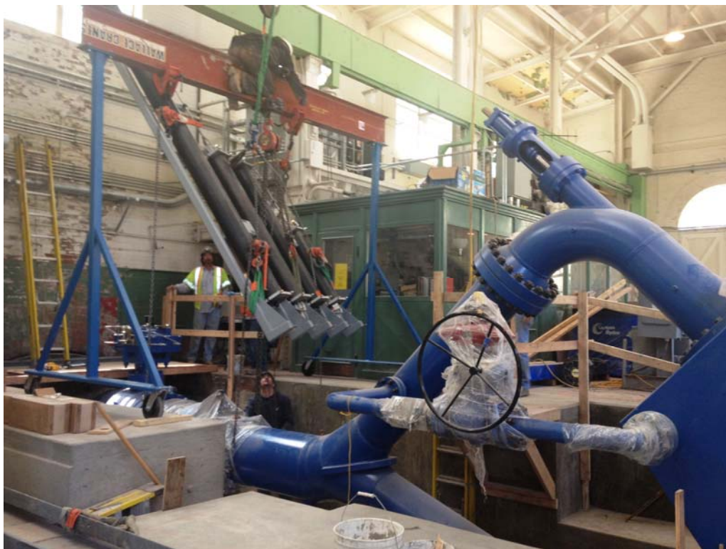
Figure 15 – Accumulator Tanks Install (5/15/12)
