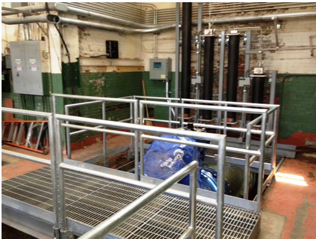
Figure 21 – Walkway & Accumulator Tanks (6/14/12)
