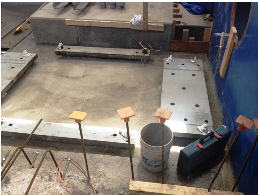
Figure 17 – Generator Sole Plates (5/15/12)
