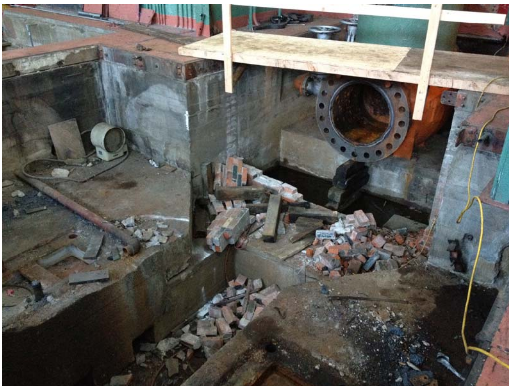
Figure 2 – Removed Turbine Piping (12/20/11)
