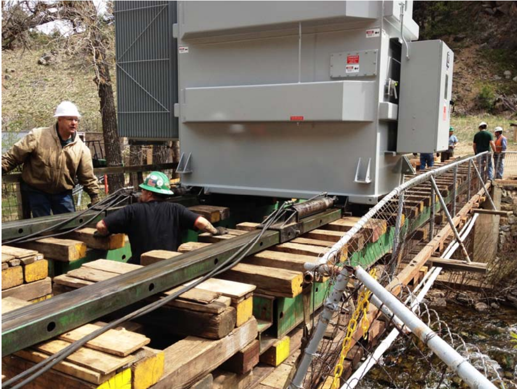
Figure 12 – Transporting New Transformer Across Access Bridge (4/19/12)
