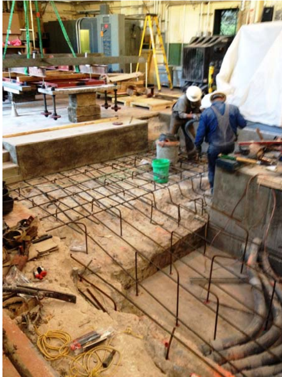
Figure 14 – Reinforcement Install for HPU & LPU Pad (5/10/12)
