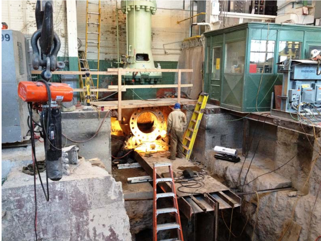
Figure 4 – Removal of Existing TIV (2/16/12)
