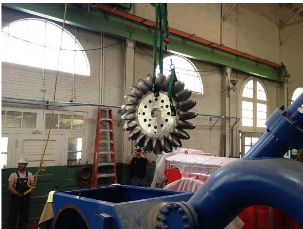
Figure 20 – Turbine Runner Install (6/14/12)
