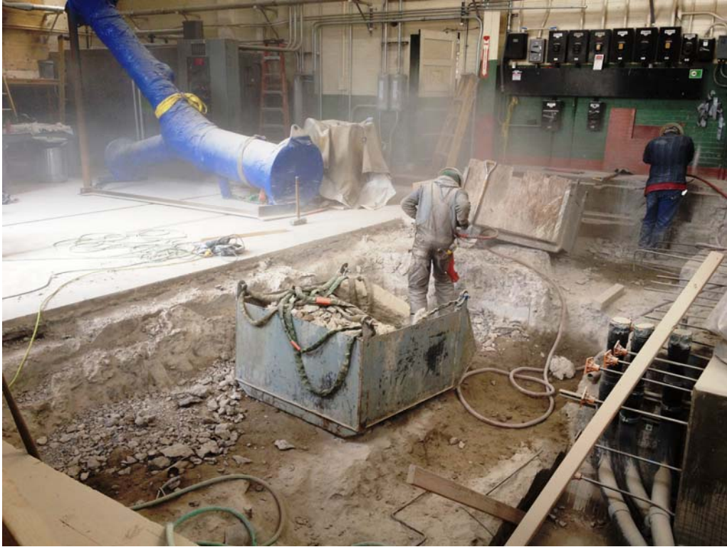
Figure 11 – Concrete Removal (4/18/12)
