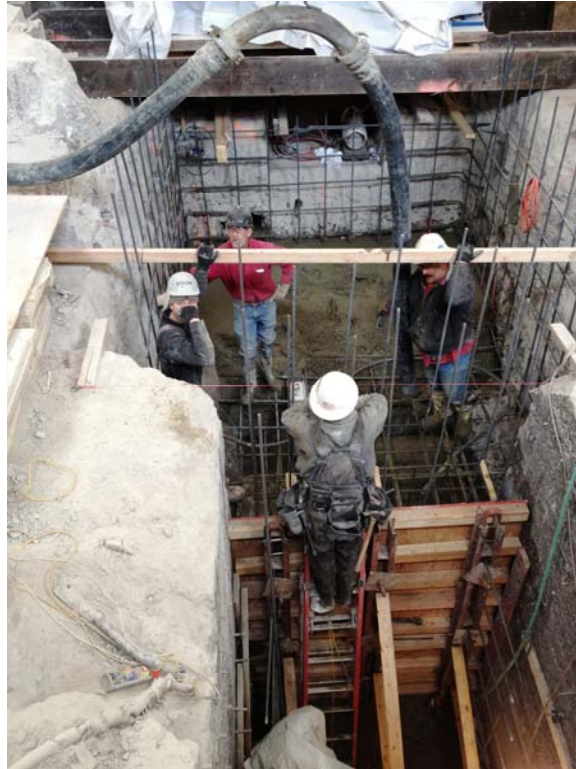
Figure 6 - Reinforcement Install for Turbine Pit (3/2/12)
