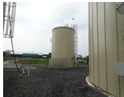
FIGURE 8: GREASE BUFFER TANK
