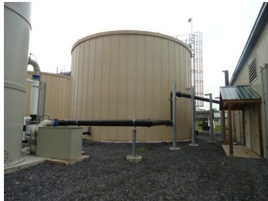
FIGURE 7: MANURE BUFFER TANK
