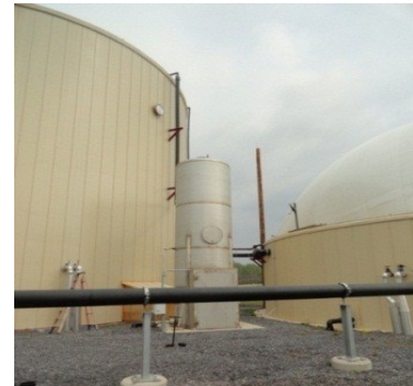
FIGURE 12: SEDIMENT RECOVERY TANK
