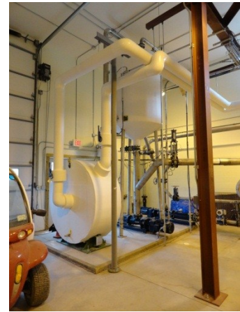
FIGURE 9: SANITATION HEAT EXCHANGER
