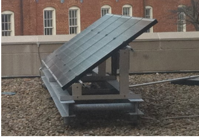
(a) Solar panels Sanyo HIP-195BA19
