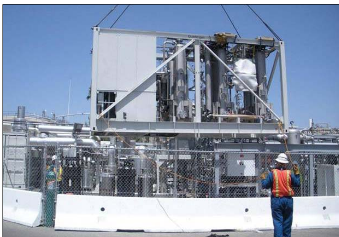
Figure 20. Installation of ADG clean-up system at OCSD.
