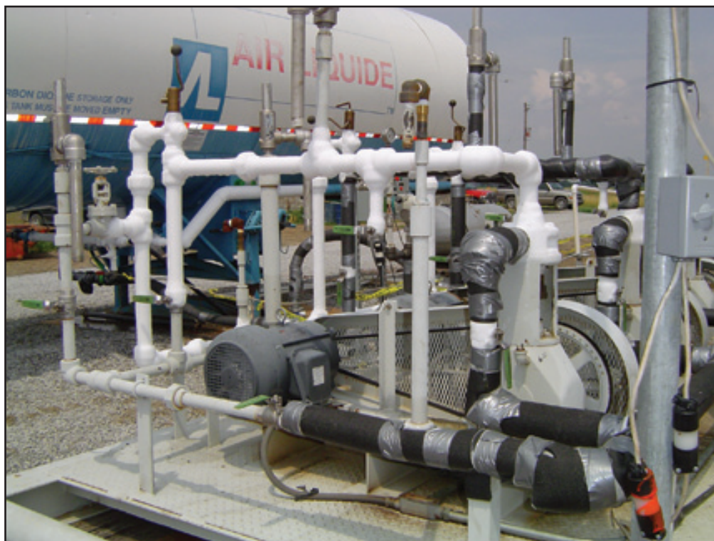
Figure 57. Main pump skid in operation (white frost on lines). Black foam insulation wrap on lines leading to pump inlet in foreground. Pump is the light gray vertical component to right; pump motor is dark gray and to the left. Black V-belt connects the pump and motor. Photograph was taken by Ray McKaskle for Trimeric Corporation.
