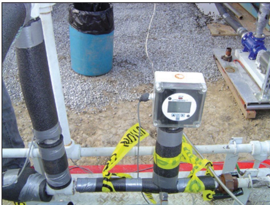
Figure 59. Flow meter on the discharge line of the main pump skid. This part of the discharge line is insulated with black foam wrap to minimize presence of two phases passing through the meter. The booster pump is in the right background. The gray pipe behind the meter is the liquid/vapor return line between the tank and pump skid. Photograph was taken by Ray McKaskle for Trimeric Corporation.
