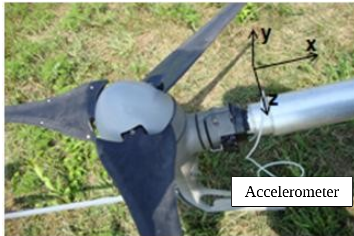
Figure 4-4: Wind turbine nacelle with coordinate system shown. The coordinate system is fixed to the tower and does not rotate with the nacelle.
