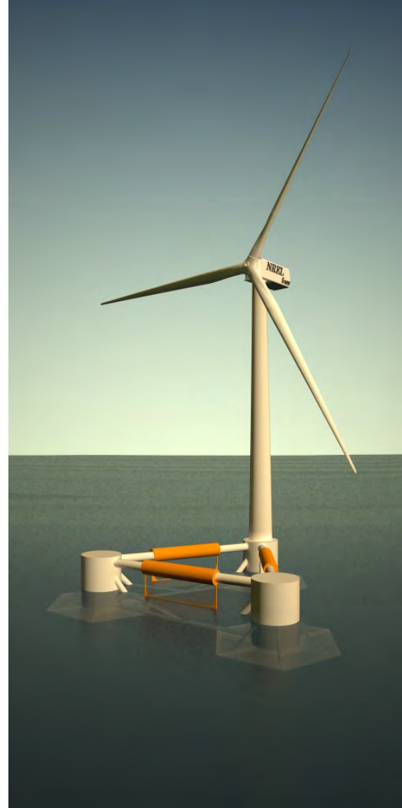
Figure 5: WindWaveFloat configuration 4, vertical oscillating plates.
