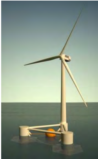
Figure 2: Single point absorber (SWEDE) integrated on the WindFloat platform.
