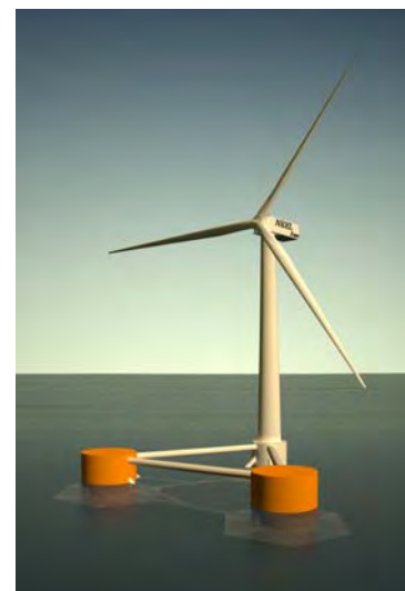
Figure 1: WindWaveFloat with two OWC Chambers
