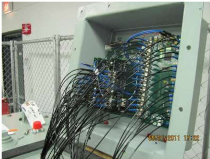
FIGURE 21: TANK STATUS AND FIBER OPTIC EXPANSION BOARDS
