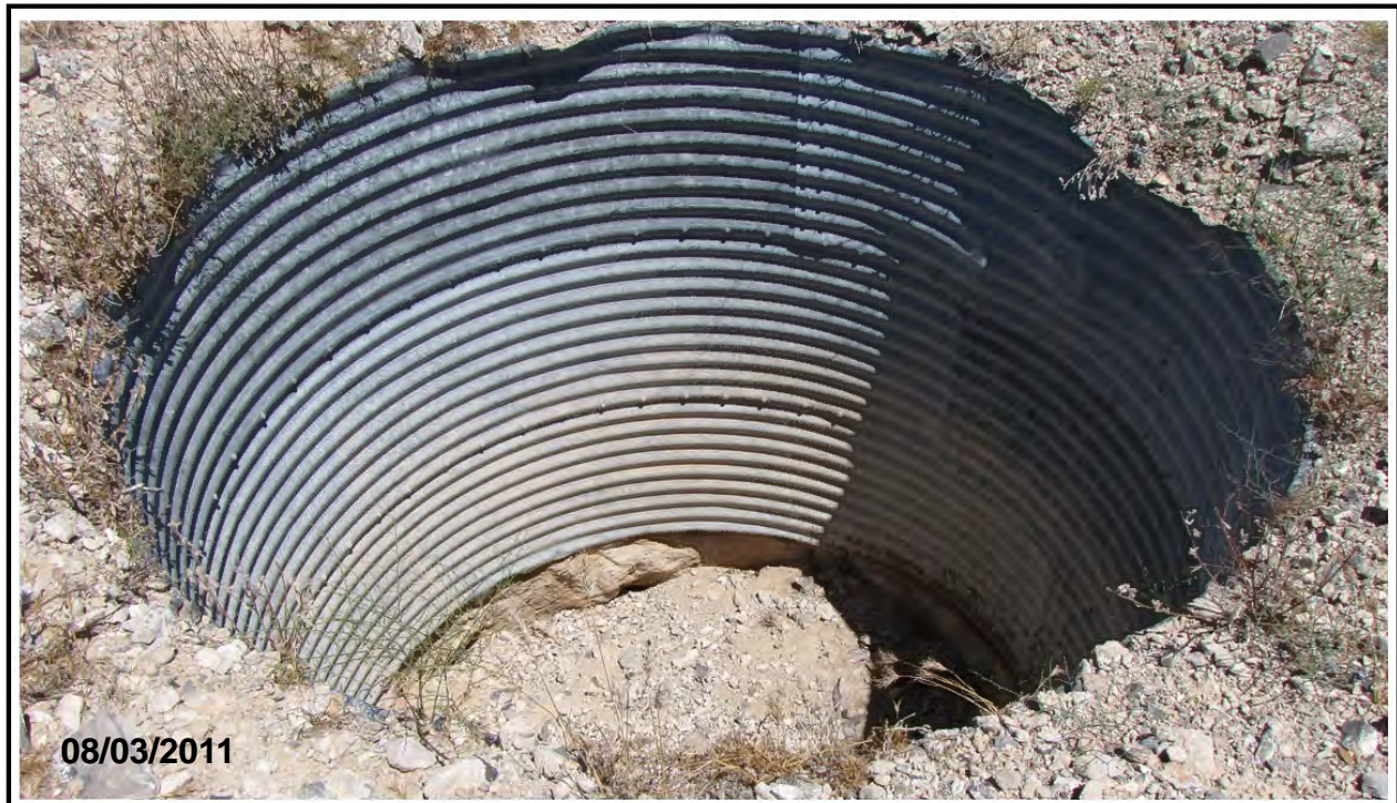
Figure 2-7 Open Disposal Borehole at CAS 00-23-02 (Dog Site)
