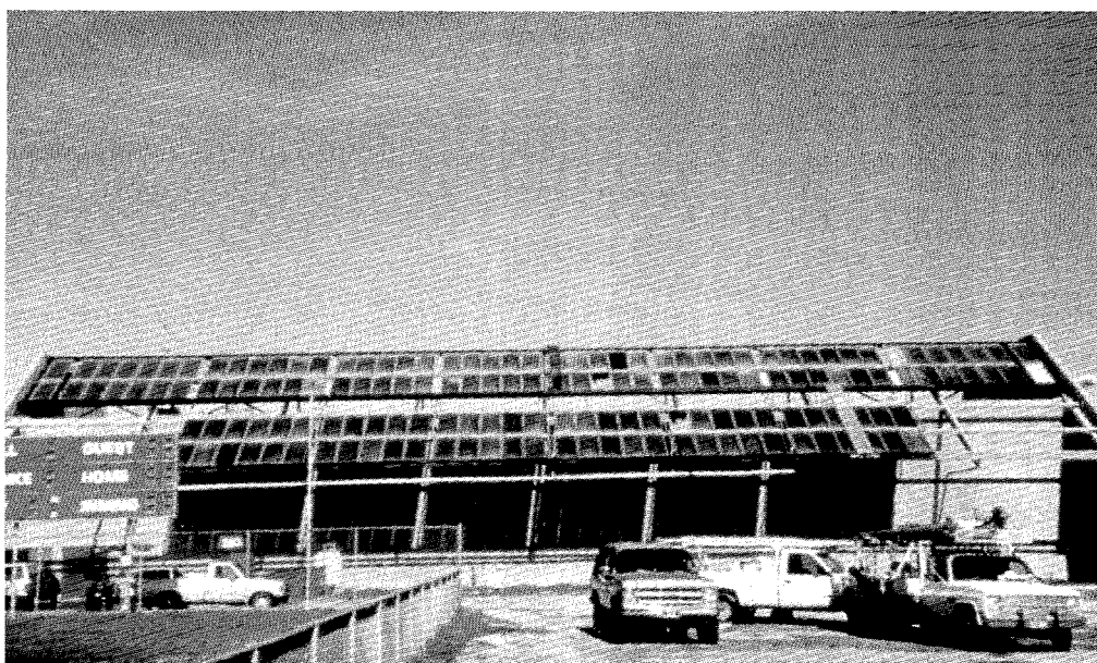
The gymnasium at Luke Air Force Base, Arizona, where solar collectors are used to heat domestic hot water, primarily for showers.
