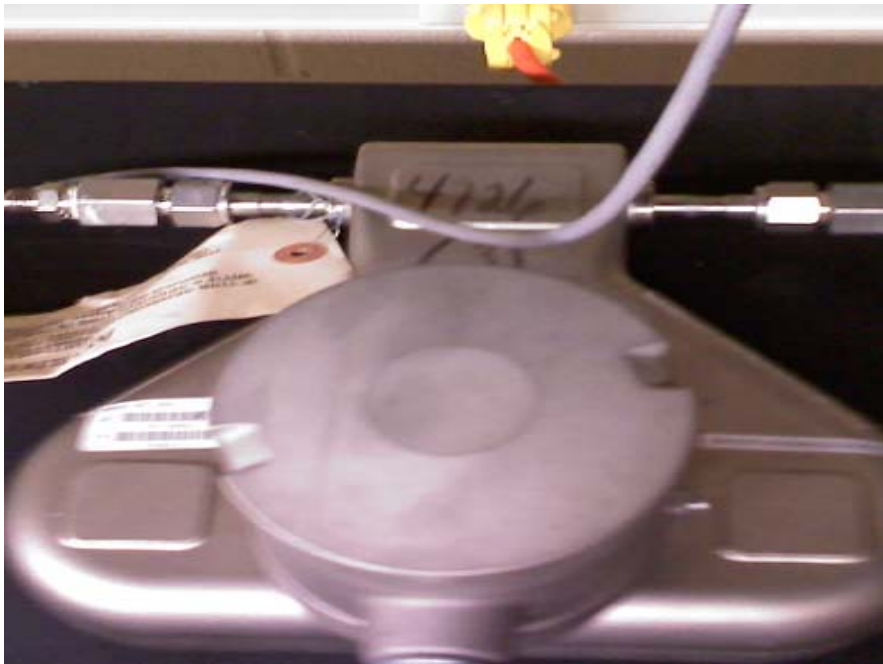
Figure 208 Rosemount CMF-010 Coriolis flow meter
