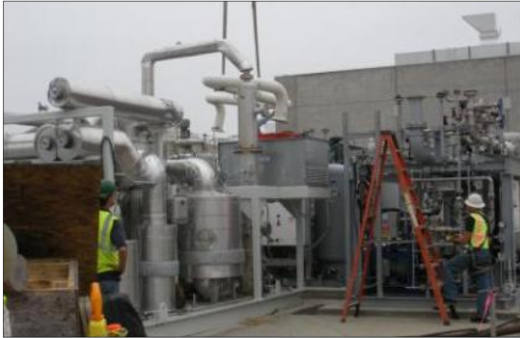
Figure 27. Installation of interconnecting piping between the DFC-300 and pressure swing adsorption system at OCSD (ground level).
