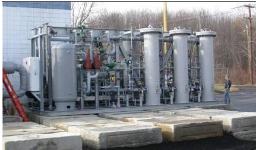
Figure 16. Pressure swing adsorption system.
