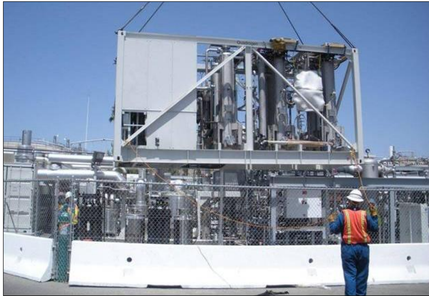
Figure 33. Installation of the ADG clean-up system at OCSD.
