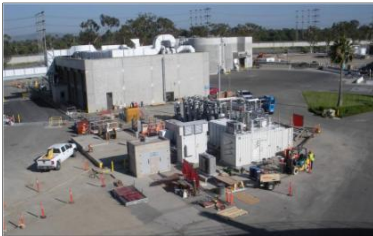
Figure 28. Installation of interconnecting piping between the DFC-300 and pressure swing adsorption system at OCSD (from above).
