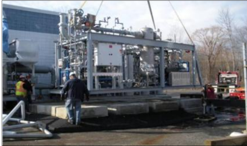
Figure 15. Hydrogen energy system compression system.
