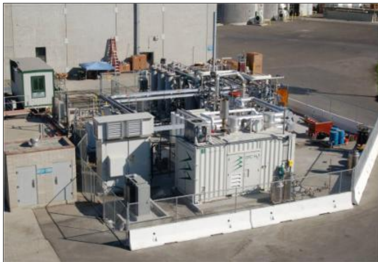
Figure 29. Installation progress at OCSD. The fuel cell is in the foreground; the pressure swing adsorption system is in the background.
