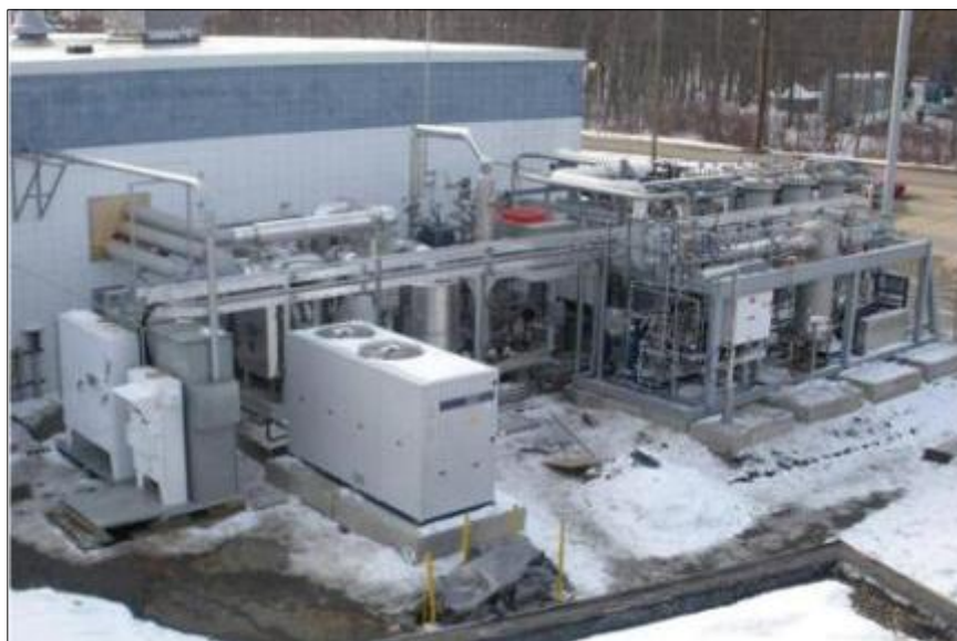
Figure 17. Hydrogen energy station installation at shop validation test.
