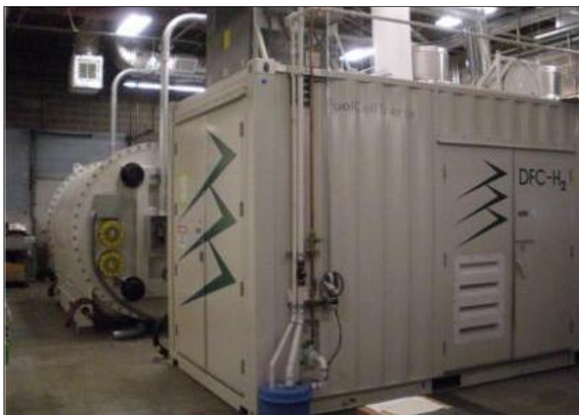
Figure 12. FuelCell Energy DFC-300 and mechanical balance of plant (MBOP).
