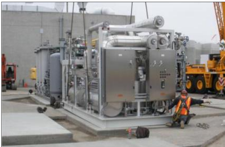
Figure 26. Installation of the anode exhaust gas skid at OCSD.
