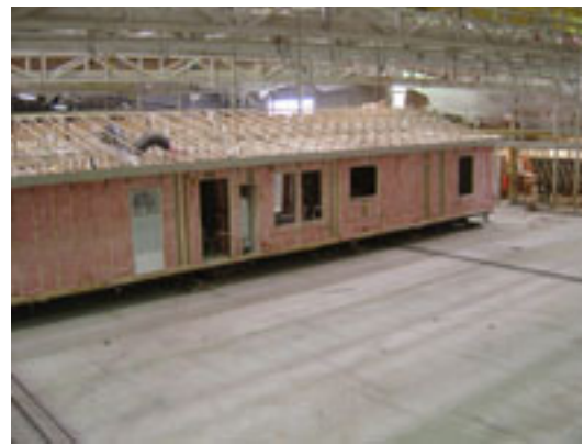
Exhibit 3.17: Roof Assembly Placed on Walls
