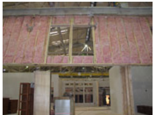
Exhibit 3.11: Lowering of Exterior Wall
