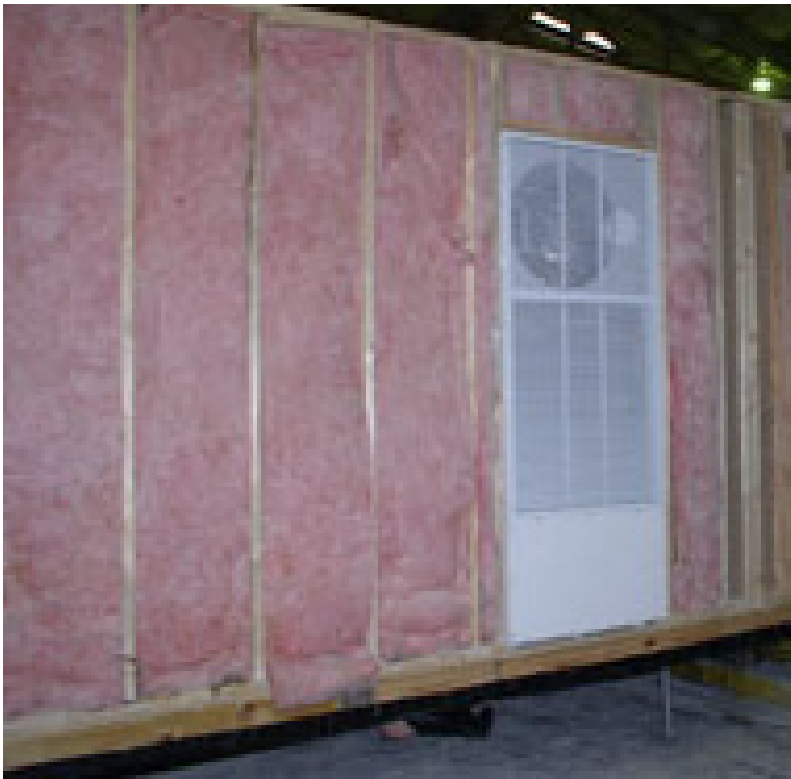
Exhibit 3.12: Final Placement of Exterior Wall with Comboflair® Unit
