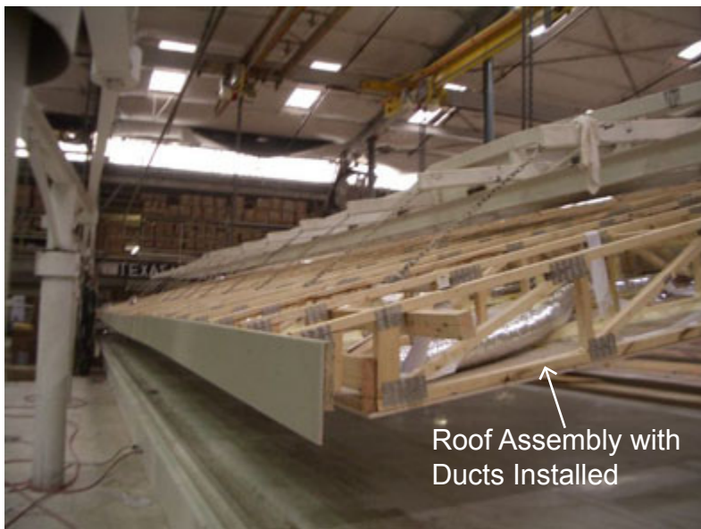
Exhibit 3.16: Roof Assembly Lifted from Assembly Table
