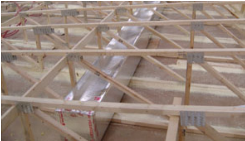
Exhibit 3.13: Trunk Duct Inserted through Roof Trusses.
