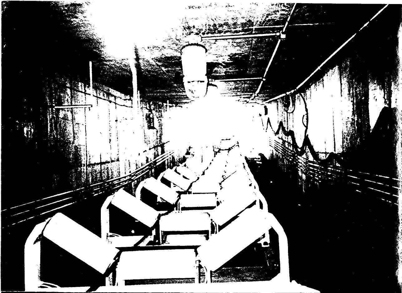
Raw coal reclaim tunnel looking from inside towards above ground opening. Conveyor belt not yet installed. Construction progress photo, April 1994.
