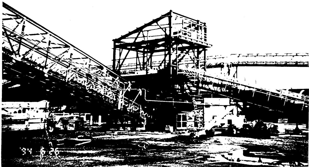
Precrusher building showing reclaim conveyor entering from the right side and plant feed conveyor exiting from the left bottom.
