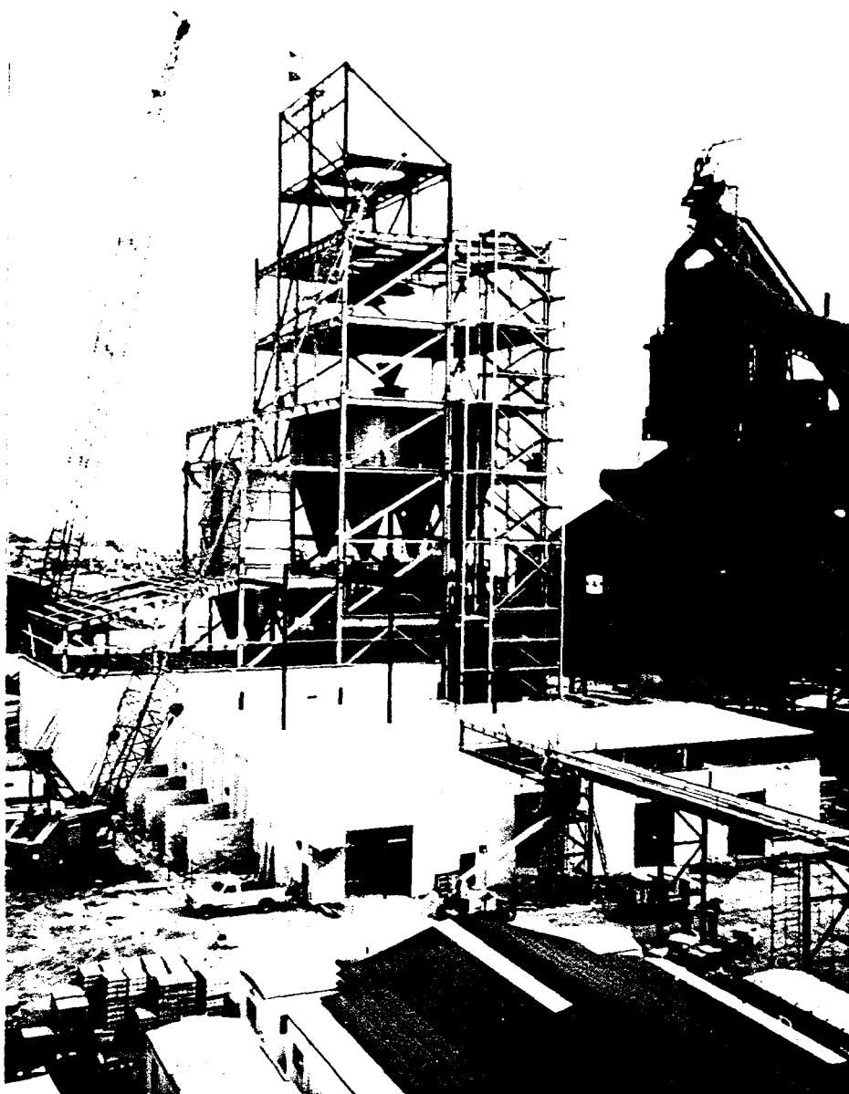
Erection of the Process Building (high structure) and Utility Building (low structure). Note the two raw coal bins and four product coal bins within the process building structure. "D" blast furnace is in the right background. Construction progress photo, February 1994.
