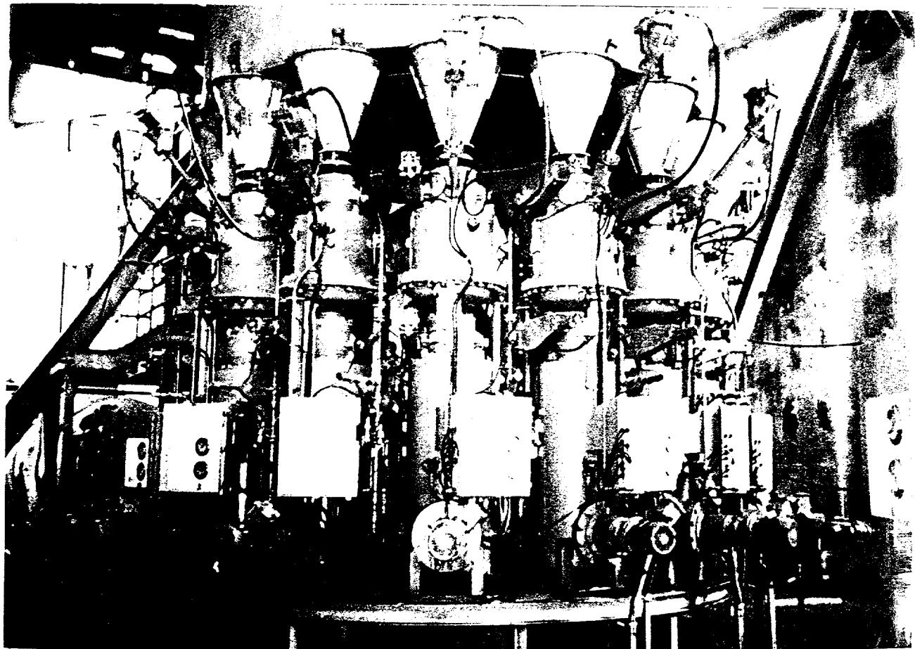
One of four clusters of fourteen coal injectors beneath the distribution bin (top of photo). Coal flows by gravity from the cylindrical-shaped distribution bin leg into the injector lockhopper. The lockhopper discharges into the injector vessel containing the motor driven screw feeder at the bottom. Construction progress photo, March 1994.
