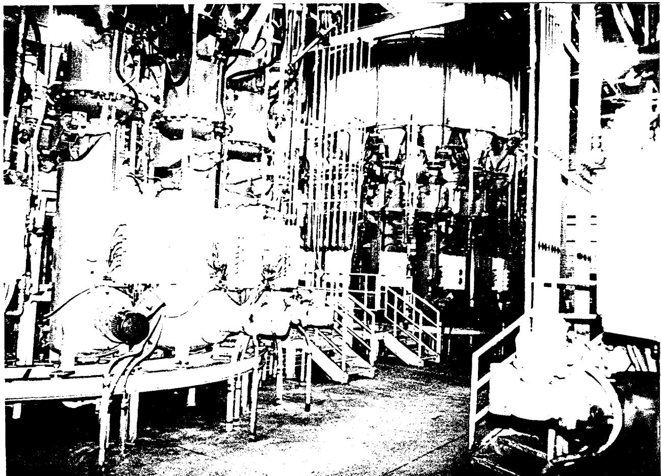
Coal injectors for "C" blast furnace beneath the distribution bin. Two clusters of 14 injectors each are required to feed each blast furnace.
