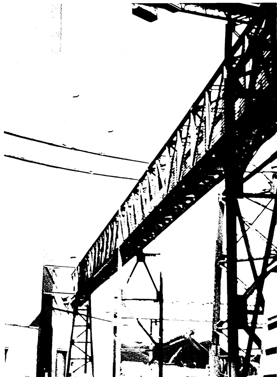
Coal injection pipe bridge from the process building to "C" blast furnace. Injection pipe bridge to "D" blast furnace can be seen in the lower background. Construction progress photo, October, 1994
