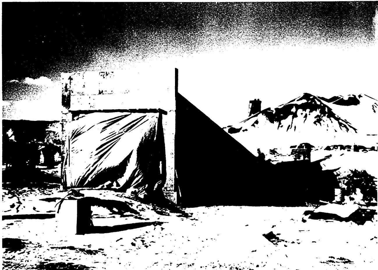
Construction of concrete underground raw coal reclaim tunnel prior to placing soil back fill material which will cover all but the tunnel opening in the foreground. Tunnel is 12' wide x 16' high x 400' long.
