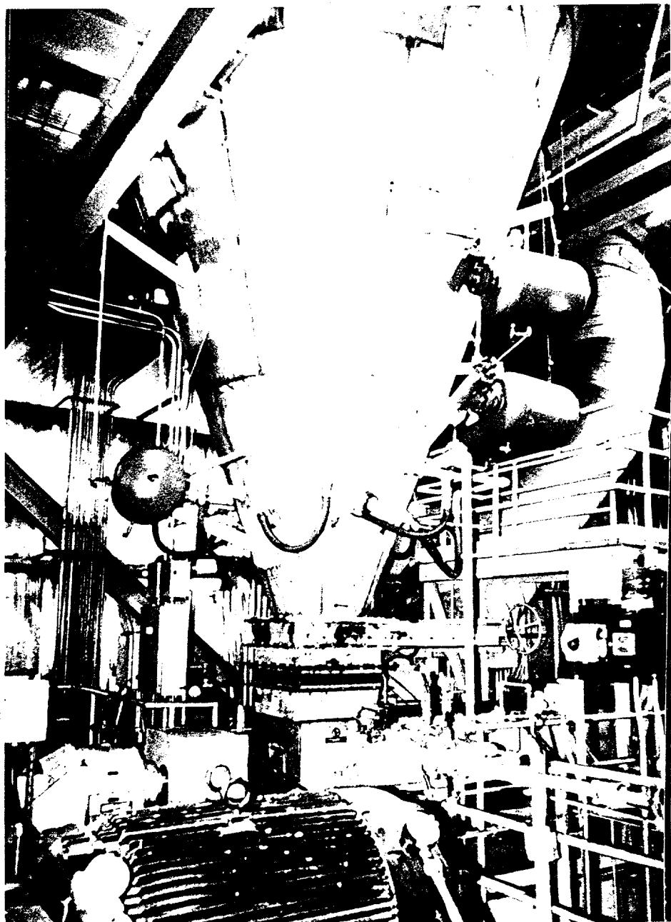
Bottom of the south 240 ton raw coal storage bin. A screw feeder takes coal from the bin bottom to the coal preparation mill.
