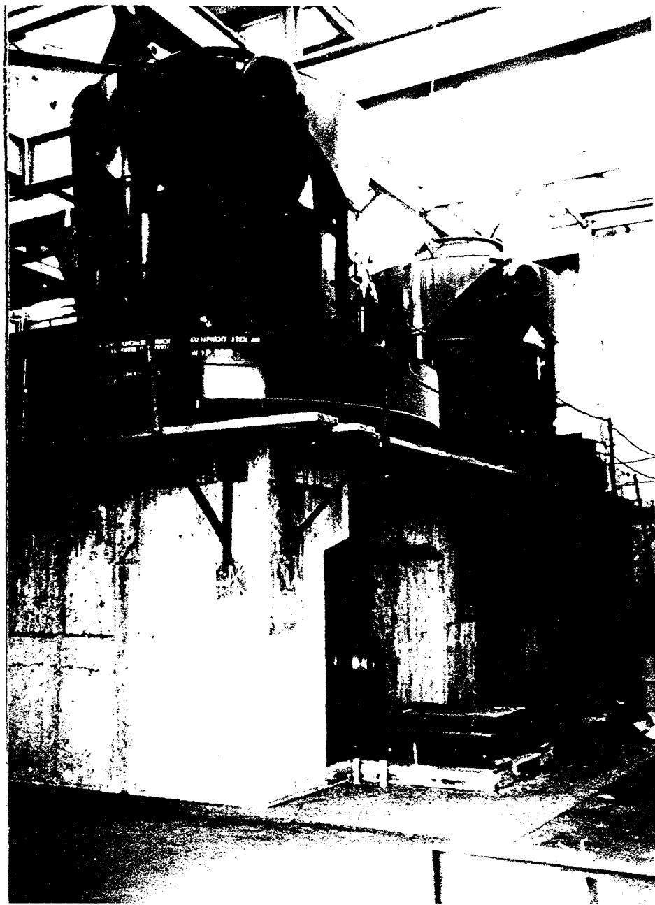
Installation of two Williams crusher/dryer mills with spinner separator on top of the mill. Gear box located between the concrete pedestals. Mill drive motor not yet installed. Construction progress photo, March 1994.
