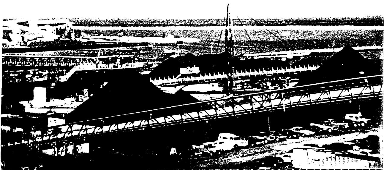
Radial stacker and raw coal stockpile area after delivery of the first train load of coal. The radial stacker is in the lowered position. Construction progress photo, September 1994.
