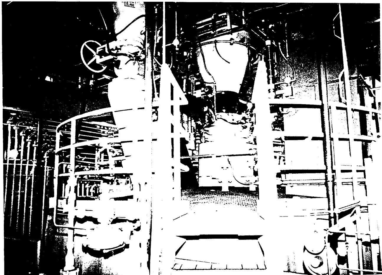
Bottom of one of four weigh bins (which takes coal from the product coal bin) discharging into the top of the distribution bin.
