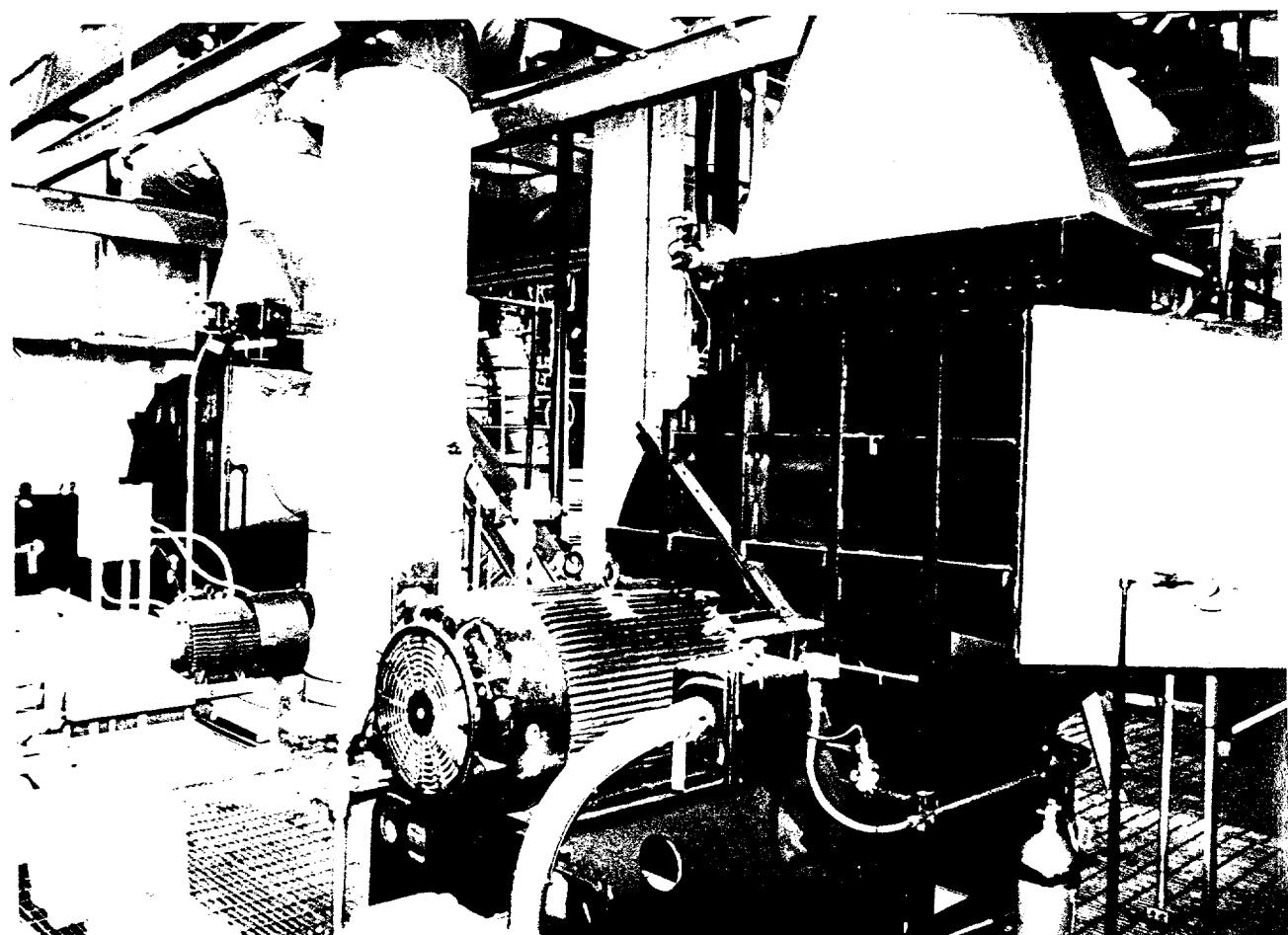
The mill system, motor driven, exhaust fan circulates a portion of the coal drying air through a dust collector located outside the building.
