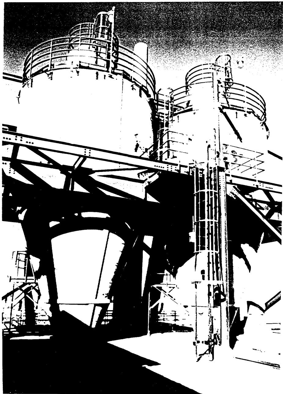
Mill system cyclone separators located on top of the Process Building. Most of the coal is removed from the drying air in these units. Coal flows from the bottom of the separator to the product coal screen inside the building. February 1995.
