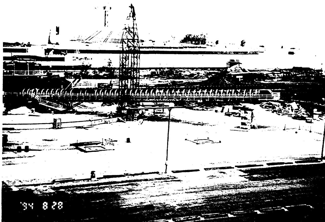
Raw coal radial stacker conveyor. Three of the four hoppers feeding coal to the underground reclaim tunnel can be seen at ground level. Construction progress photo, August 1994.
