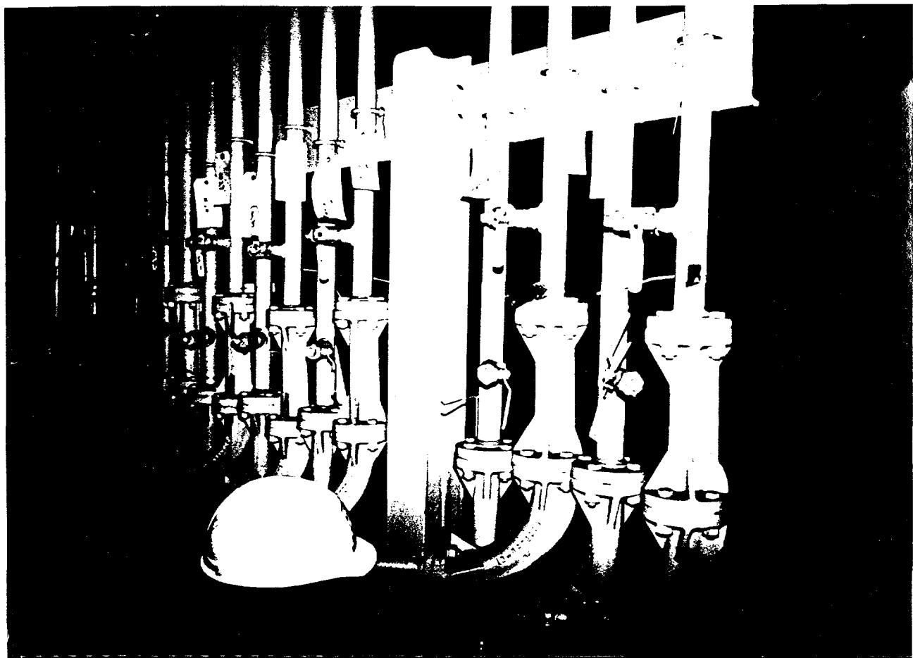
Coal injection piping inside the process building. Special hardened pipe elbows are necessary at each change in coal flow direction.
