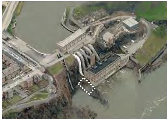
Figure 2-2 Existing School Street Power House. The dashed box indicates the planned location for installation of the Alden turbine
