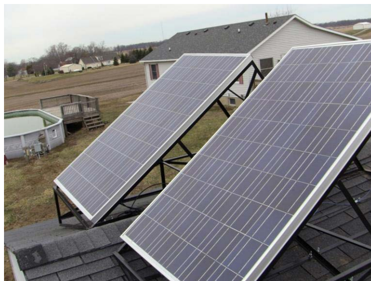
Figure 28: Solar panels used in solar irrigation system.
