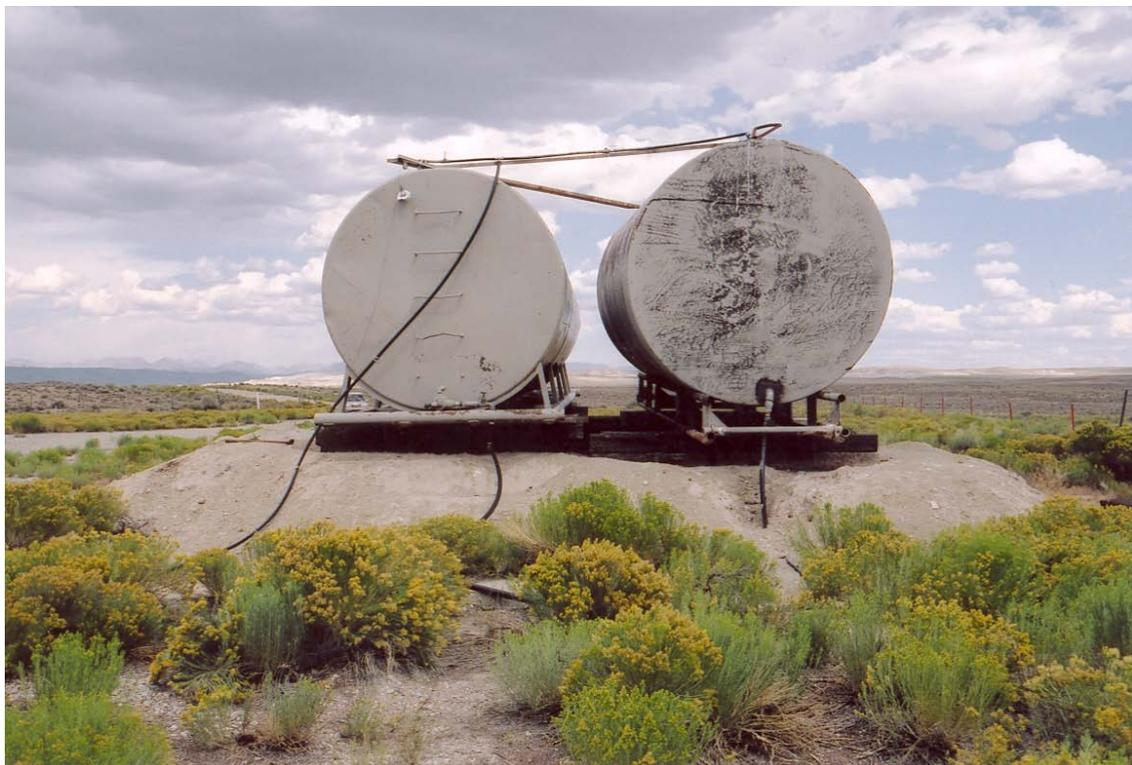
Figure 3.26-14. Tanks from the Wagon Wheel Project reused as water tanks (photo taken August 10, 2003 on file at Desert Research Institute).
