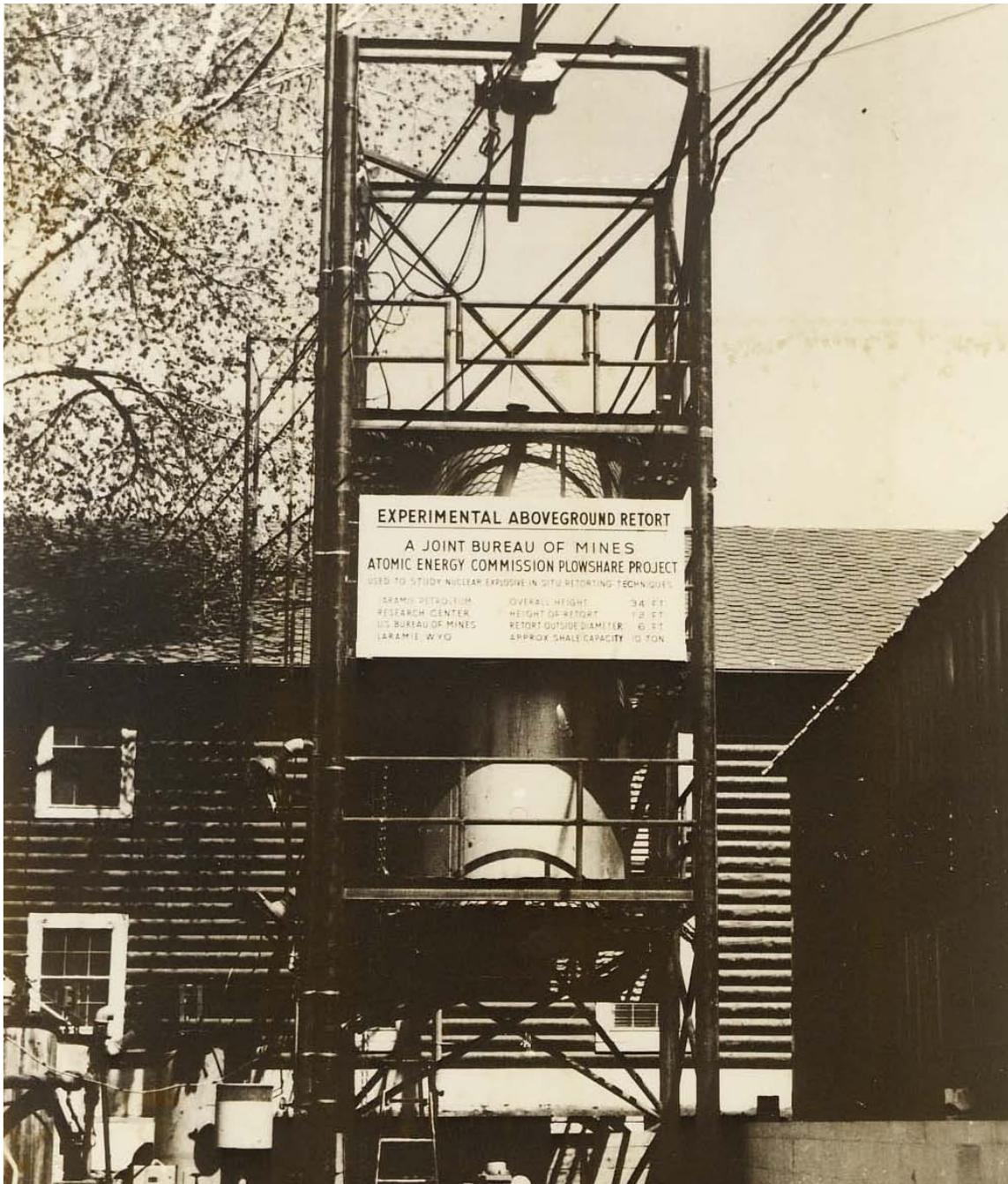
Figure 3.25-4. An experimental above ground retort for the Plowshare Program (Lawrence Livermore National Laboratory n.d., Negative No. GLB-666-4764).
