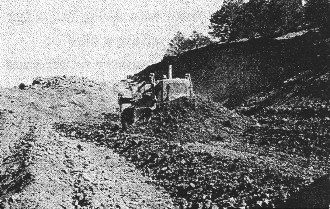
Figure 3.23-8. Railroad Relocation Cut #2 being excavated after the double row-charge detonation (from Lattery 1974, Figure 7a).
