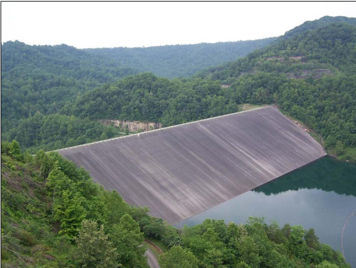
Figure 3.17-6. View of the upstream concrete face of the dam for the R. D. Bailey Lake Project. The spillway is located on the northern (far) side of the dam ([http://en.wikipedia.org/wiki/R.\\_D.\\_Bailey\\_Lake](http://en.wikipedia.org/wiki/R._D._Bailey_Lake), last accessed August 2008).
