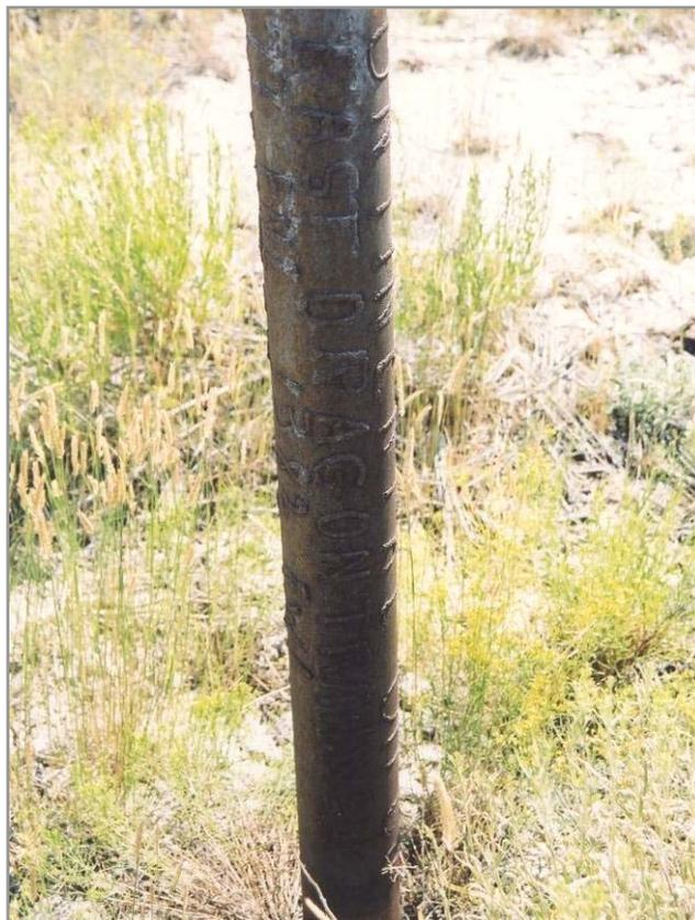
Figure 3.4-8. Close-up of welding on Project Dragon Trail study well DT-B (photo taken August 2005 on file at Desert Research Institute).
