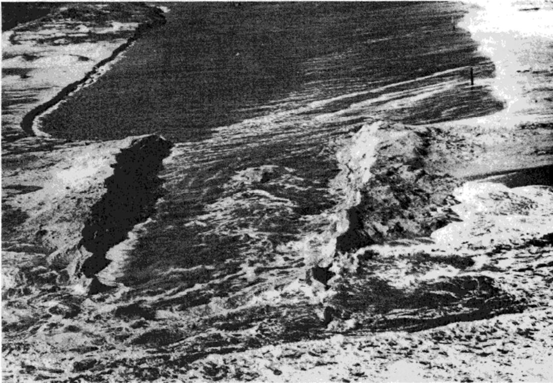
Figure 3.5-4. Post-detonation photograph of the Drum Inlet channel with a view toward the Core Sound showing the dredged channel in the background and explosive excavation in the foreground (from Snell and Gillespie 1973, Figure 17).
