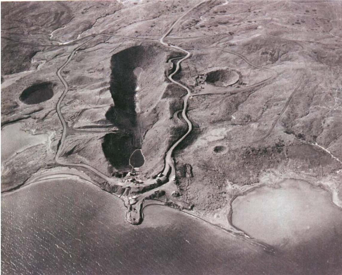
Figure 3.15-8. The Pre-Gondola III trench after the detonation of the Phase II row charge. Works crews are shown preparing the emplacement holes for the final explosive series to make the connection to the reservoir c. Sept. 1969 (Lawrence Radiation Laboratory, U.S. Army Engineer Nuclear Cratering Group 1969, no figure number).
