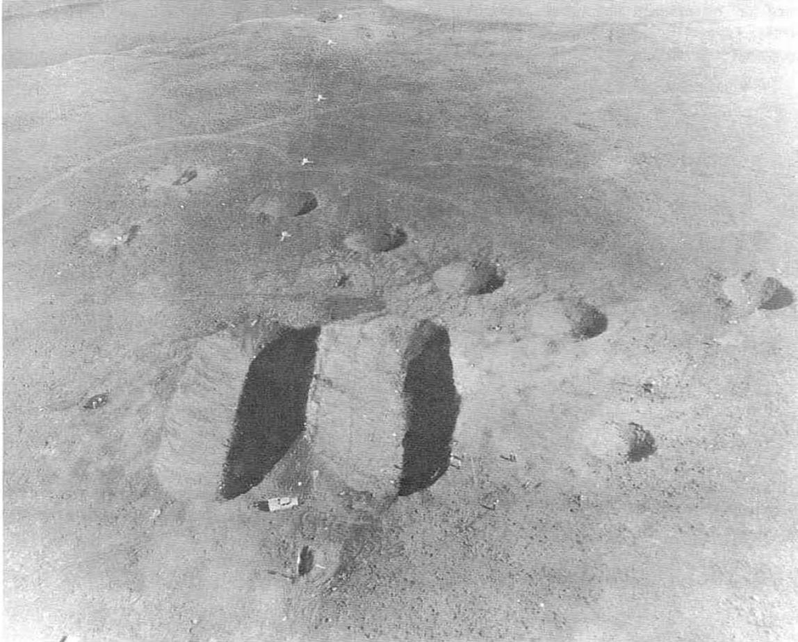
Figure 3.15-7. Aerial view of the Project Pre-Gondola III, Phase I triple-row shot before the detonation of the center row. The surrounding individual craters are from the associated 1-ton calibrations shots (Cress et al. 1970, Figure 7).
