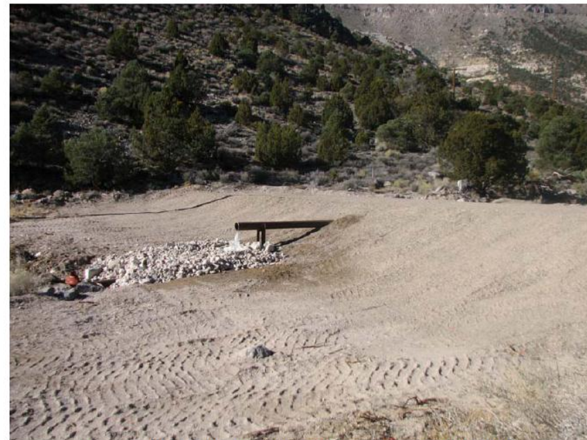
Photograph 3. Overflow Pipe at Upper Berm (12/11/2008)
