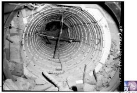
Figure 7: Photos of damage levels after detonation for Hard Hat 1
