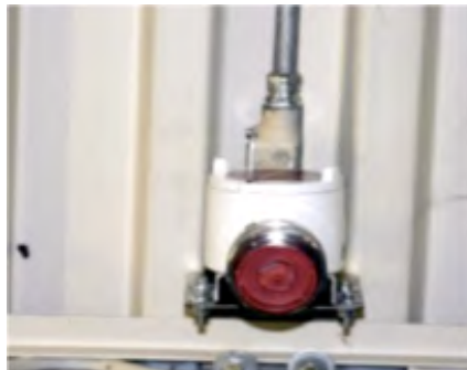
Hydrogen Gas Sensor (mounted at highest point in the ceiling)
