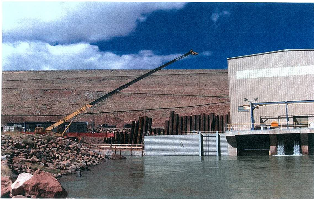
Coffer dam complete and Rio Chama allowed to backwater adjacent to power house. Abiquiu Dam in background - 4 Mar 2010.
