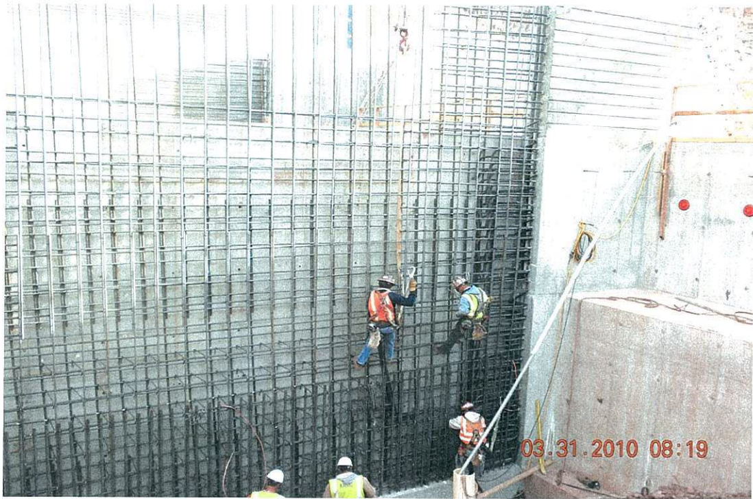
Construction of new power house - 31 Mar 2010. Cofferdam to the right in photo.
