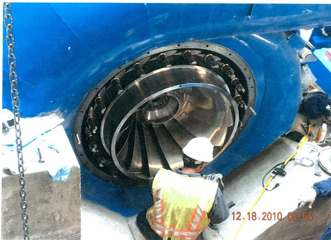
Installing new turbine runner - 18 November 2010.
