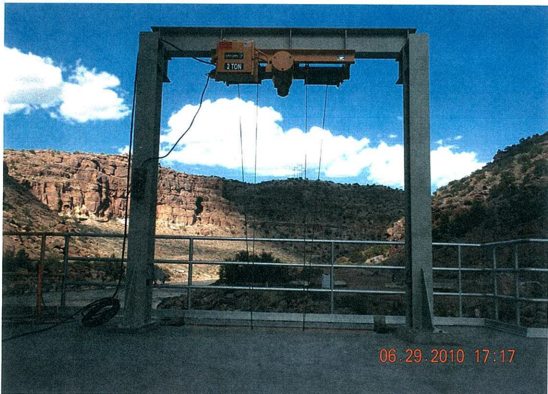
Finished installation of new draft tube gate hoist. Looking downstream - 29 June 2010.
