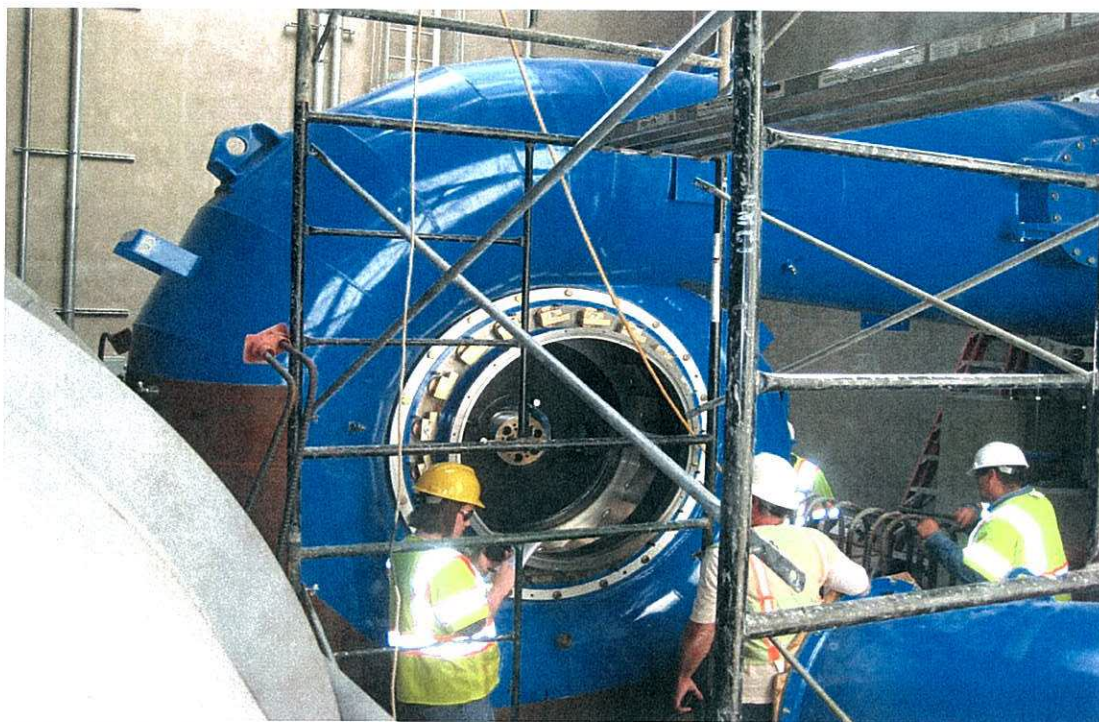
Installing and checking level of new turbine - 20 October 2010.
