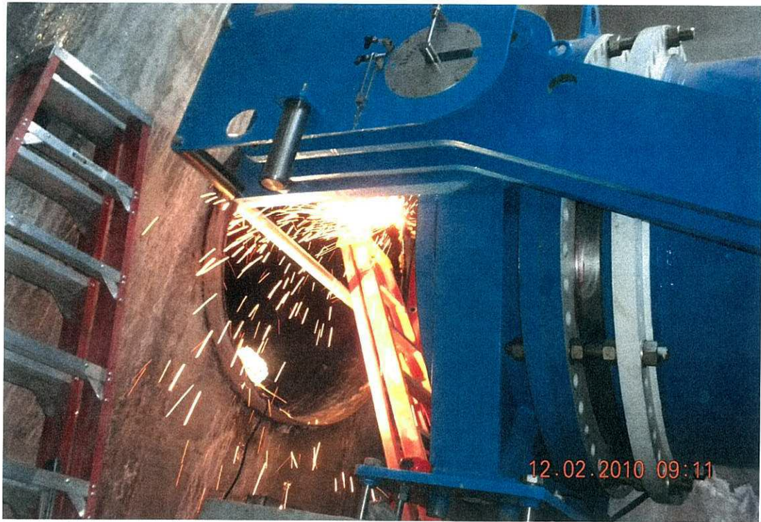
Preparing penstock connection upstream of turbine inlet valve - 2 Dec 2010.
