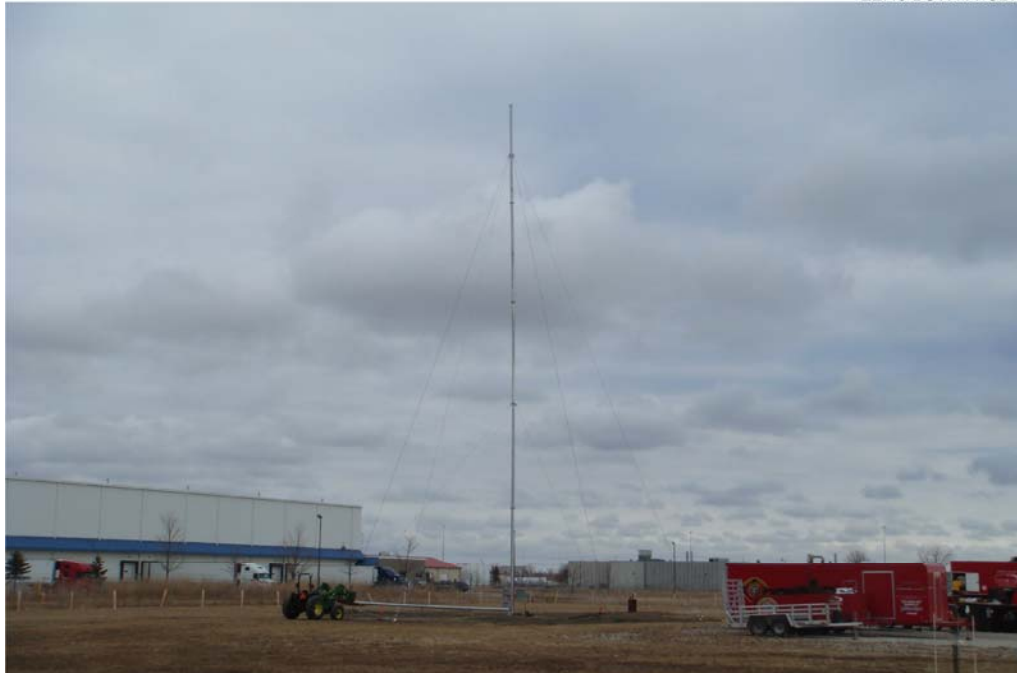
Figure 7. Tower fully erected and guy wires tensioned.
