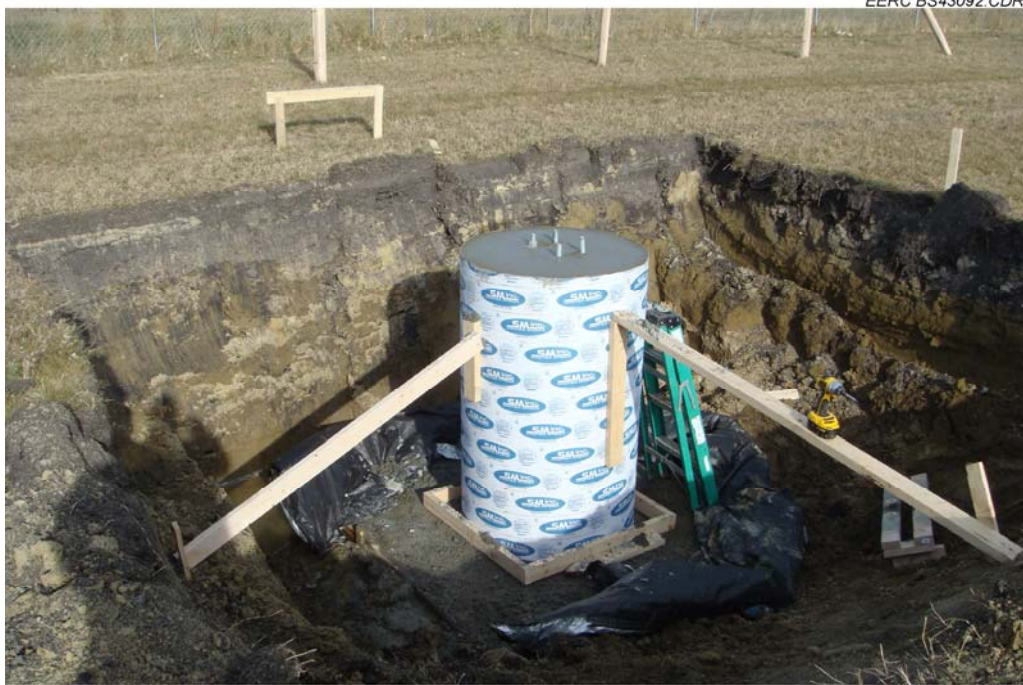
Figure 3. Winch anchor foundation.
