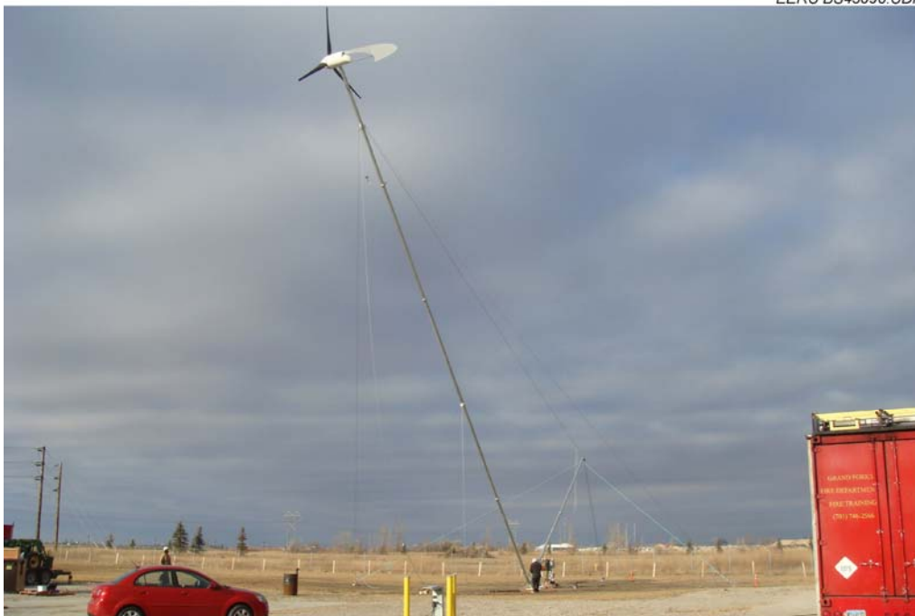
Figure 9. Fully assembled wind turbine being erected.
