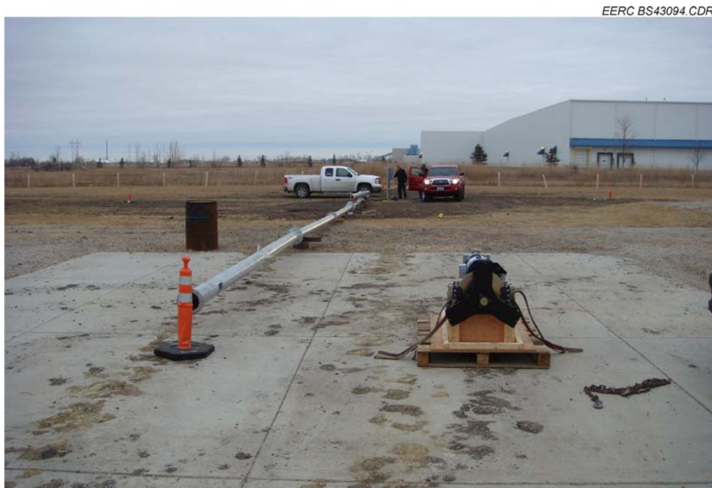
Figure 5. Tower and gin pole assembled.
