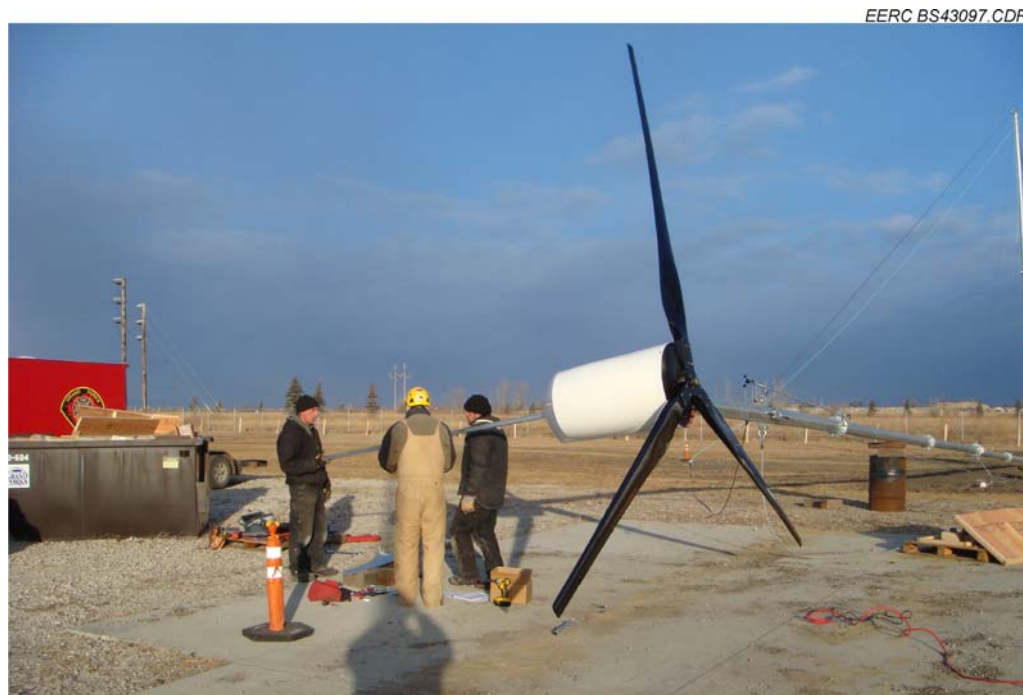
Figure 8. Mounting the turbine, blades, and tail.
