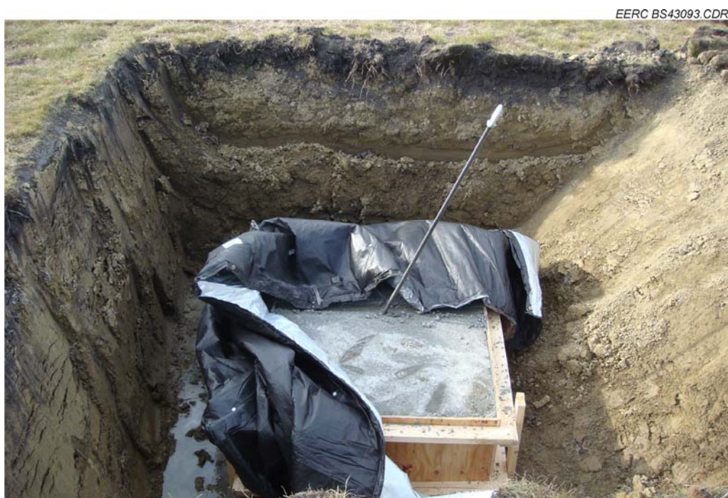
Figure 4. Guy anchor foundation.
