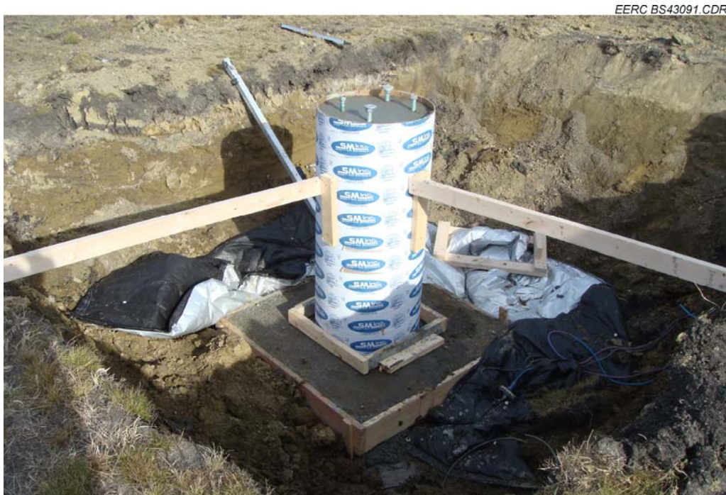
Figure 2. Tower base foundation.
