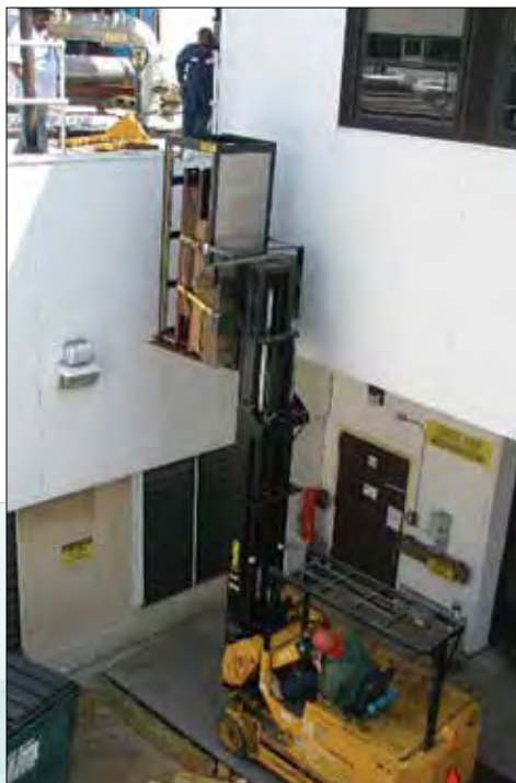
Carefully lowering the old 3,000-pound plate supply
