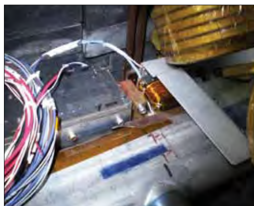
New trim magnet in the lab (top) and installed in the Booster-to-X-Ray extraction line (bottom)
