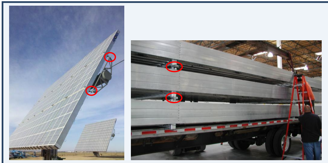
Figure 7-3: The MegaModule's central welded frames serve two purposes, (1) to fasten each MegaModule to the sun-tracking structure and (2) for securing the MegaModules together for truck-transport.
