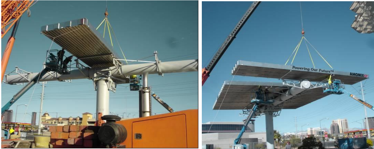
Figure 10-2. MegaModule being installed on the first 7700 system.
