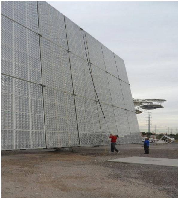
Figure 10- 9. Amonix-designed extended pole brush used to wash lenses.
