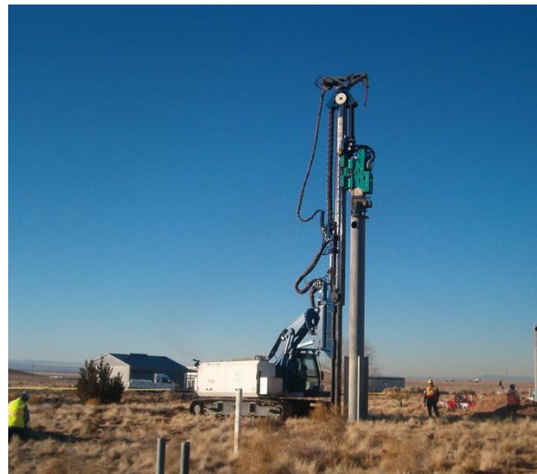
Figure 10-8: Vibratory installation of pedestal.
