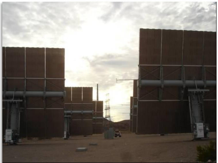
Figure 9-3: Gen 1 tracking systems installed at Southern Nevada Water Authority.
