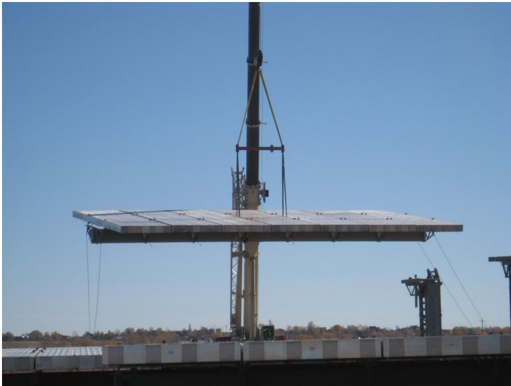
Figure 10-7. Lifting seven MegaModule array to drive head.
