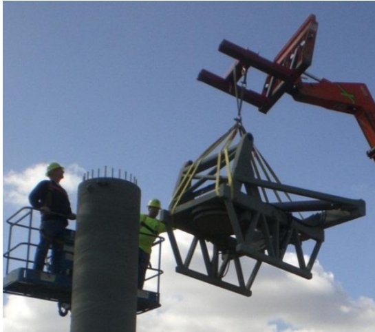
Figure 9-8. New drive head installation at City of Industry, CA.
