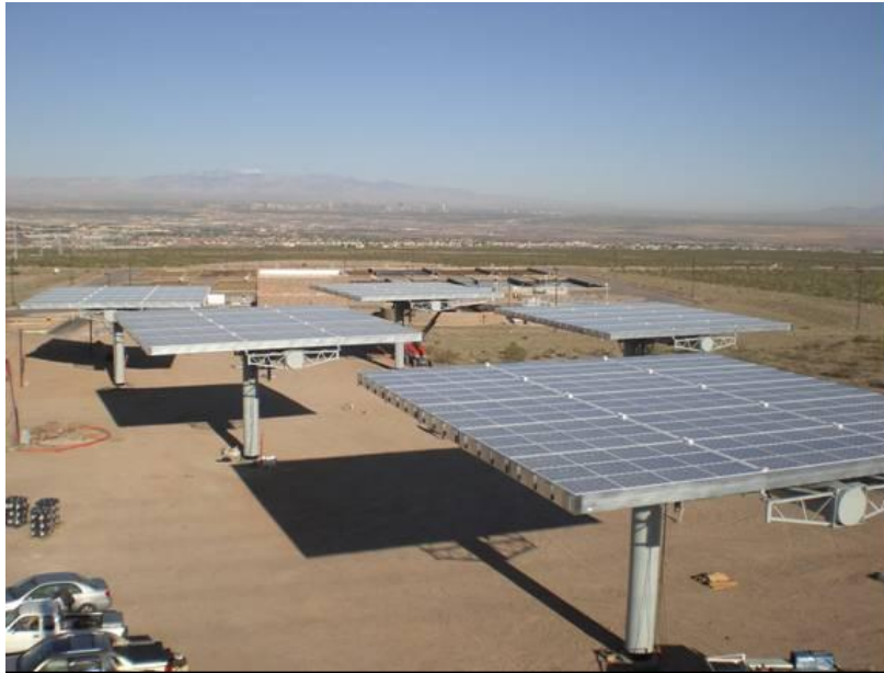
Figure 7-6. Amonix 7500-series systems installed at Southern Nevada Water Authority. These MegaModules incorporated a less expensive corrosion-protection design and easier-to-install fasteners.
