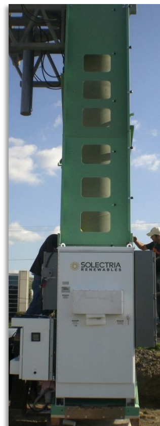
Figure 10-5 Service module electrical side.
