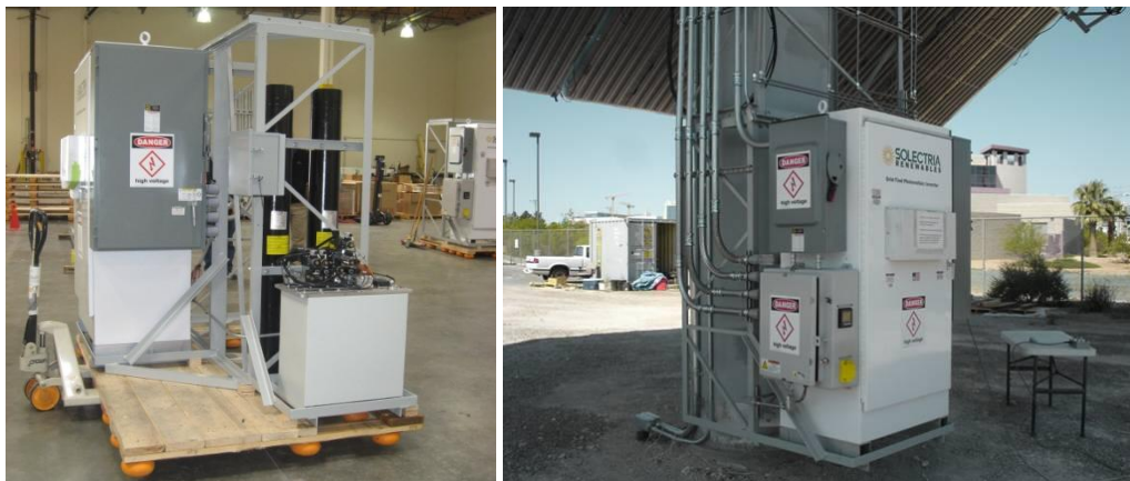
Figure 10-3. Service module assembled in factory and installed on the 7700 system at UNLV.
