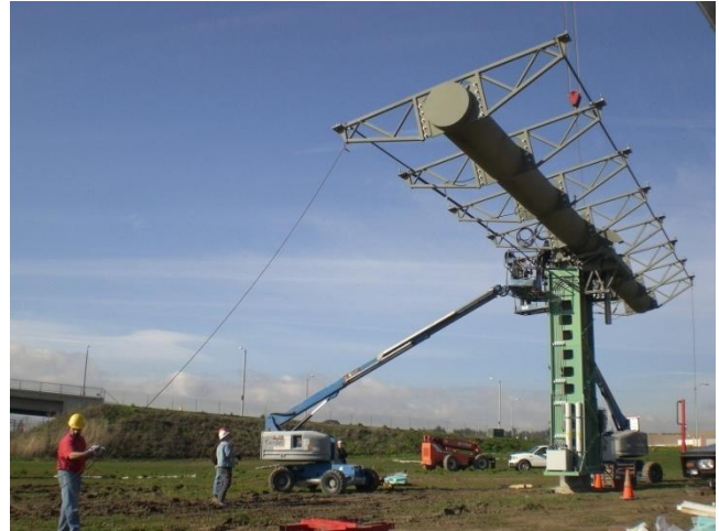
Figure 9-9. Installation of cost-reduced torque tube, pedestal and outriggers at City of Industry, CA.
