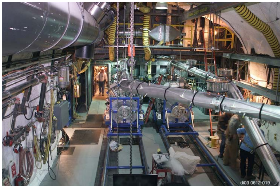
Figure 6. View of the 05 Drift tunnel expanse with the Cygnus IVAs shown in the center. The barrier is located in the background. The Coaxial Transmission Lines are also prominent.
