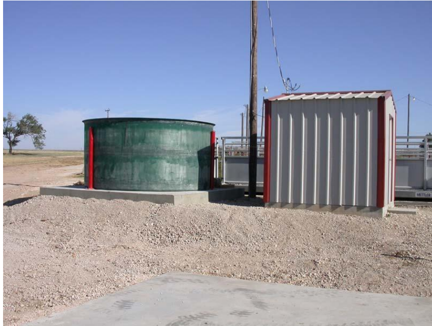
Figure B.1. Finished concrete pads and water-supply tank for anaerobic digesters at the Bushland Texas AgriLife Research/ARS feedlot.
