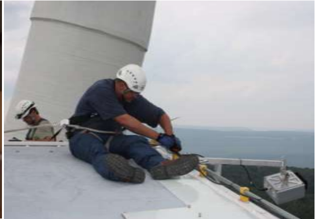
Attaching devices to a safety rail on the top of the turbine nacelle (M. Baker, Bat Conservation International).
