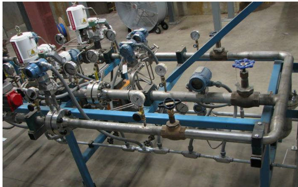
Figure 17. Photographs of the liquid oxygen tank and evaporator (top), and the valve skid (bottom)
