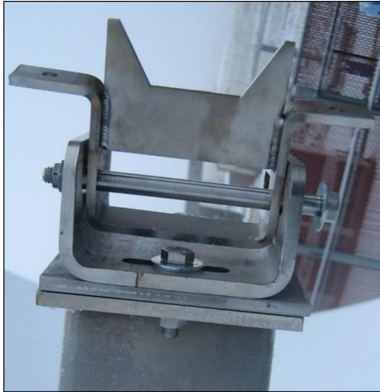
Figure 35: Tube support saddle
