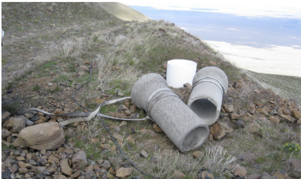
Figure 56. Two 4-foot concrete culvert sections were pulled up the mountainside to the access road (azimuth north).
