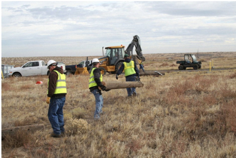
Figure 29. The poles were cut in half and removed from site 45BN826 manually, keeping heavy mechanized equipment off the site altogether (azimuth east).
