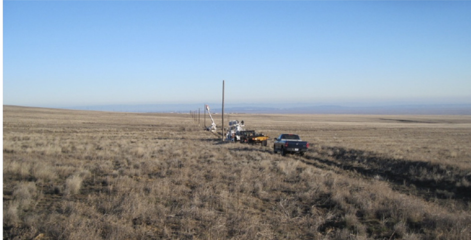
Figure 41. The method of pole removal switched to a single-file system so vehicles remained on the road (azimuth north).
