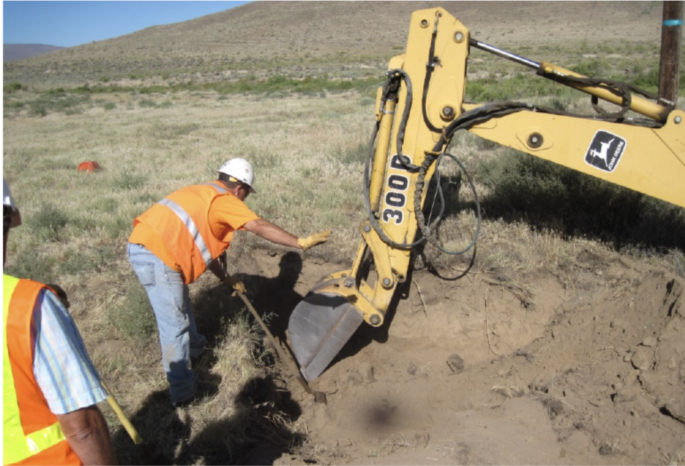
Figure 26. The well crew began decommissioning activities by exposing the well head (azimuth west).
