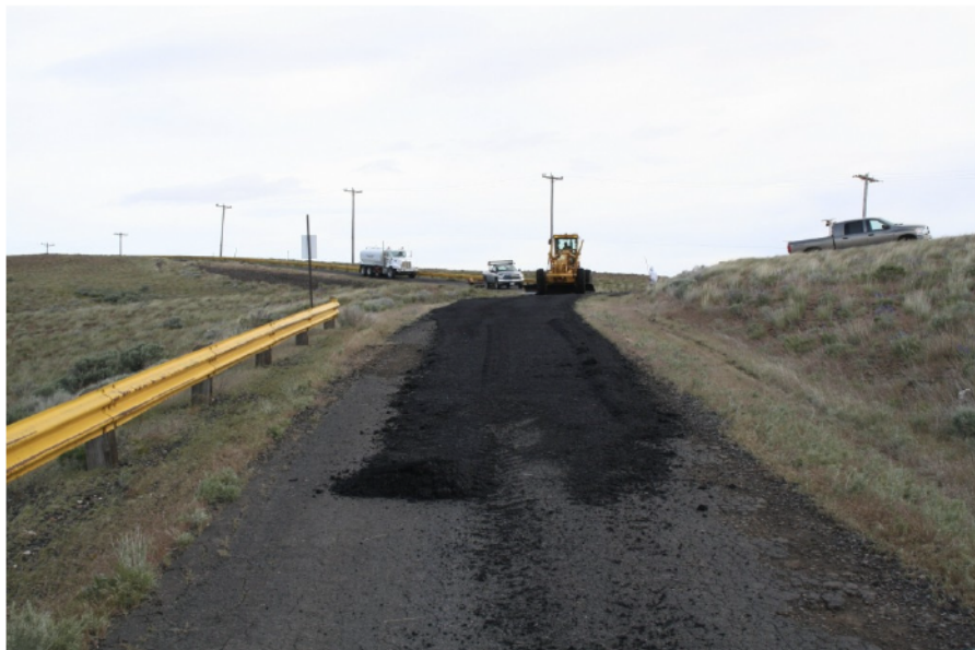
Figure 35. Crews repaired the crumbled edge of the pavement (azimuth north).
