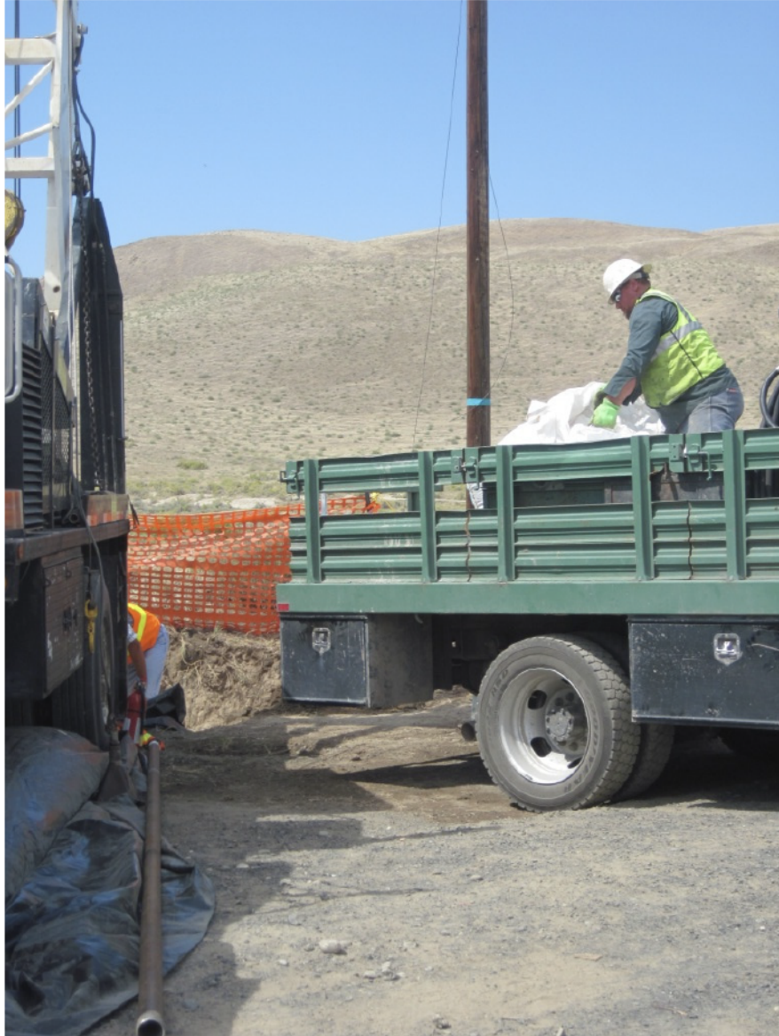
Figure 27. Well decommissioning crew members extracted vertical supply pipes from the well location, and radiation technicians cleared them for contamination (azimuth west). Decommissioning activities concluded by filling the void left by the extracted pipes with sand.
