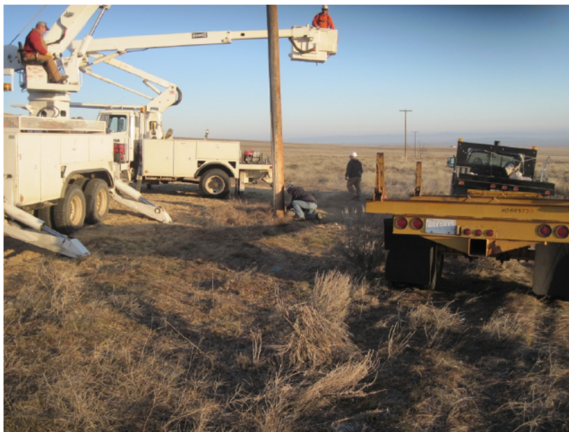
Figure 38. Pole removal activities on Lower ALE (azimuth northeast).
