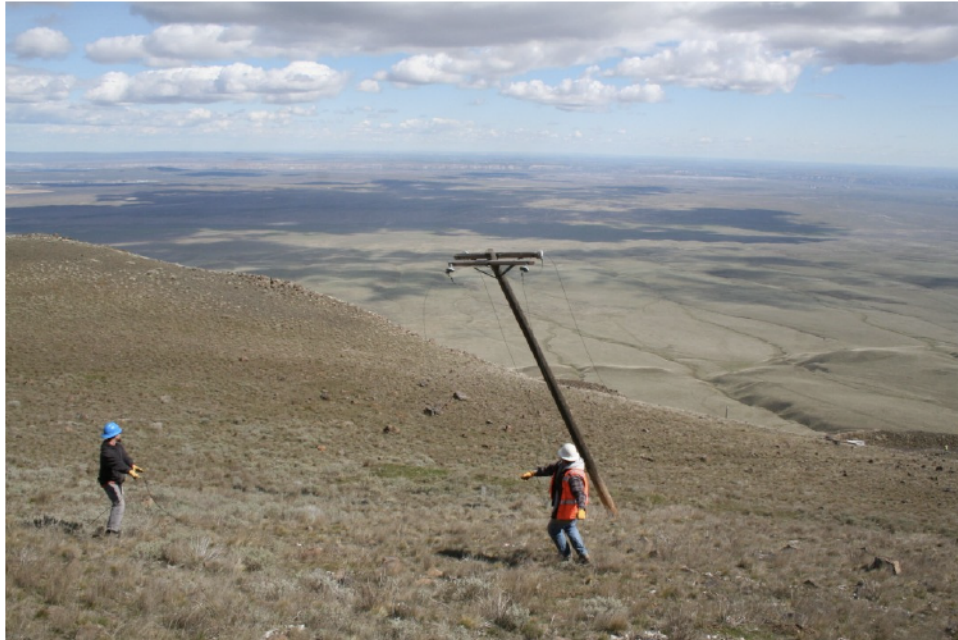
Figure 51. Ropes were used to control the landing of each pole (azimuth is east).
