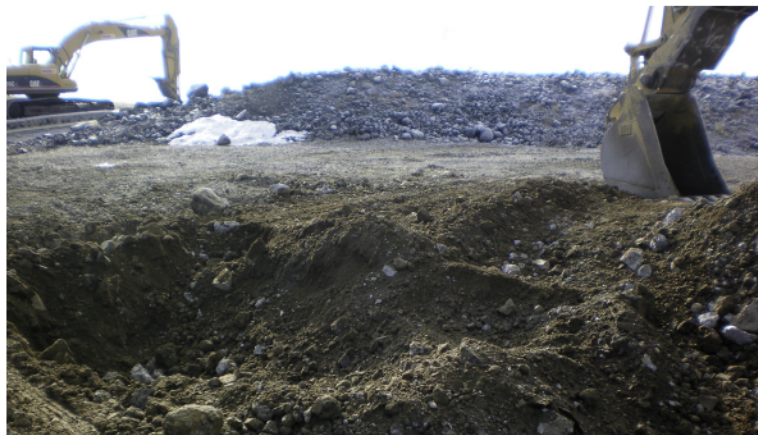
Figure 10. The trackhoe bucket (upper right) filtered concrete rubble from the ground (azimuth west).
