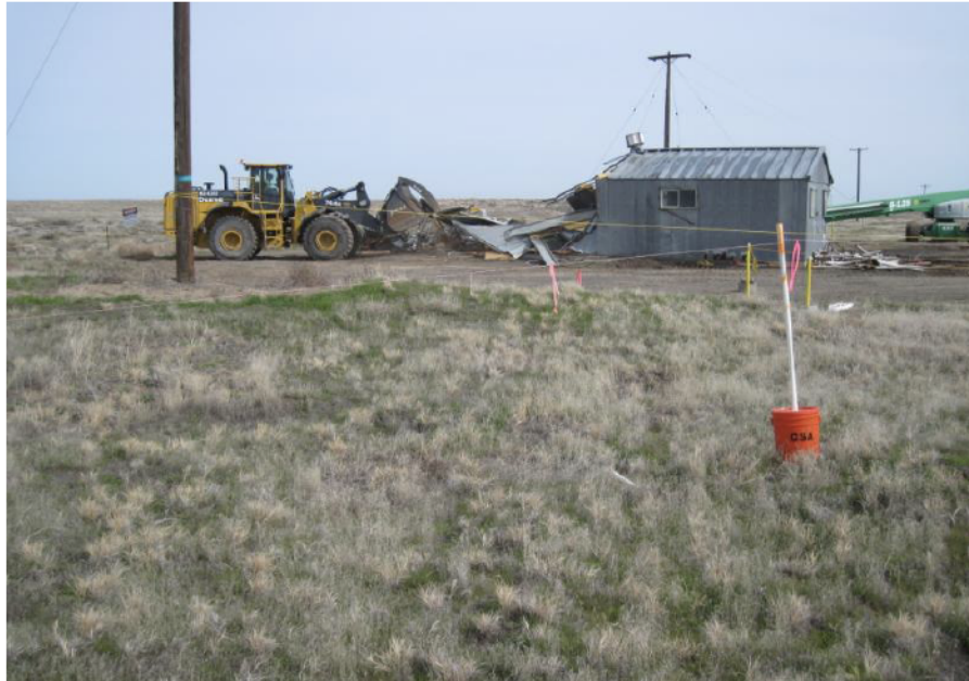
Figure 24. A wheel loader demolished the 646 Building (azimuth east).
