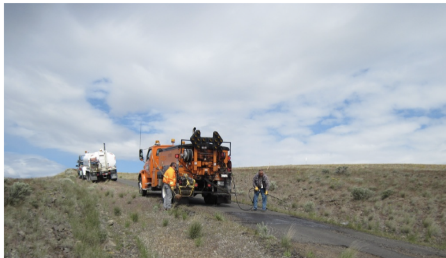
Figure 31. The paving crew prepared to deposit asphalt over the top of a damaged section of roadway (azimuth north).
