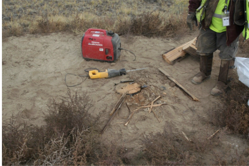
Figure 30. The poles were cut flush with the ground surface using equipment that would not leave a residue behind, such as chainsaw bar oil (azimuth north).
