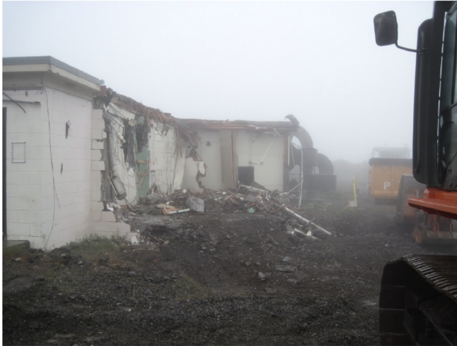
Figure 19. Demolition on the southeast corner of the 6652-C Building (azimuth north). The southeast and northwest corners of the building already had been demolished.
