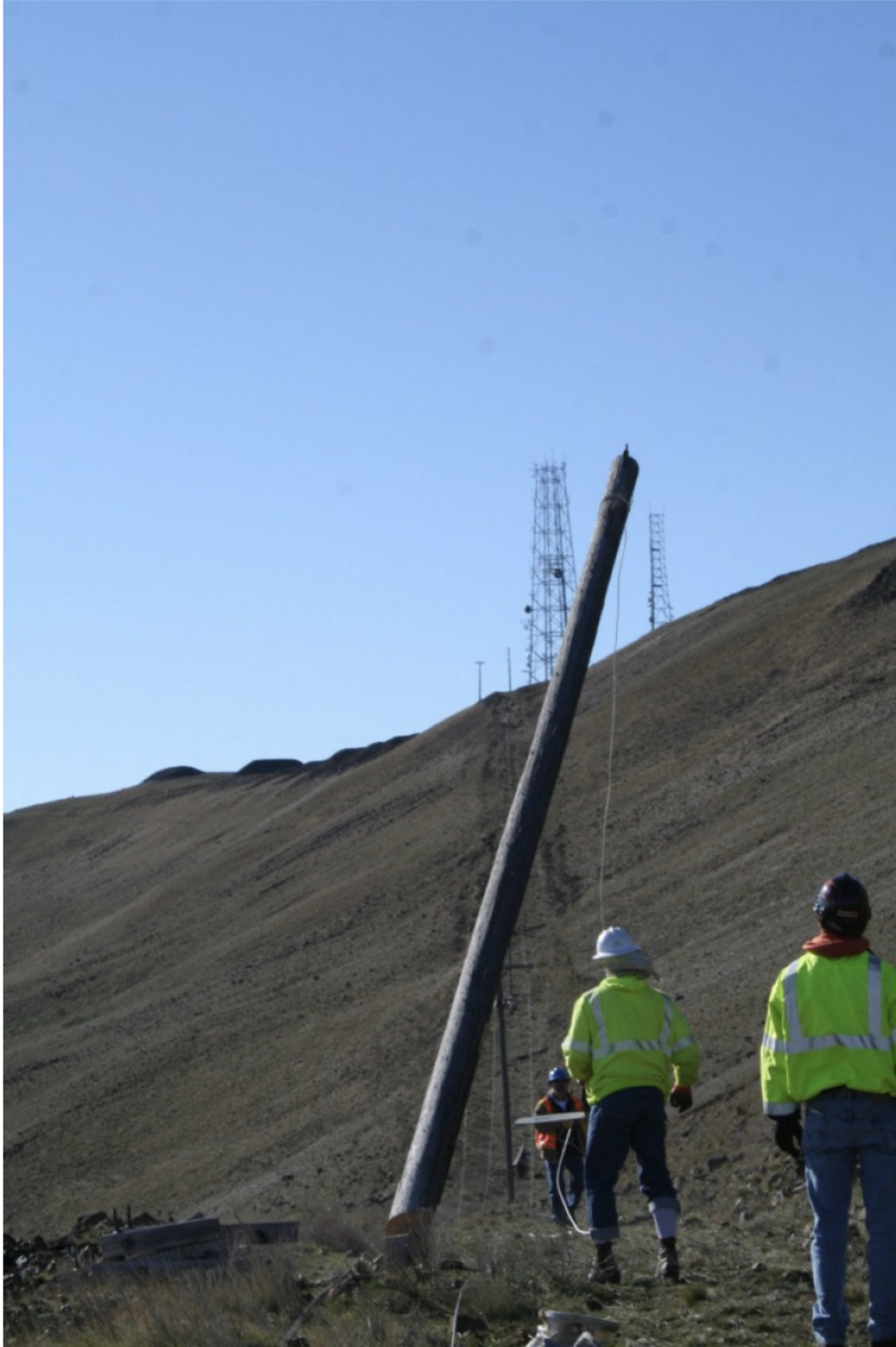
Figure 49. Power poles on the power line access road were felled on that road (azimuth southwest).
