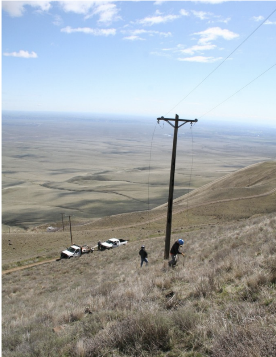
Figure 50. A lateral power pole line ascended the north side of Rattlesnake Mountain. The removal of each pole represented a unique tactical issue (azimuth southeast).
