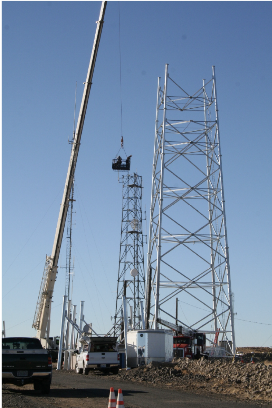
Figure 8. Two cranes worked to erect the new CCCF tower (azimuth north).
