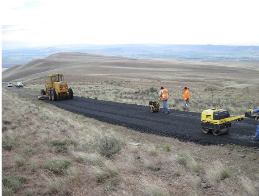
Figure 32. The paving crew spread and compacted a large linear patch over a section of the roadbed (azimuth southwest).
