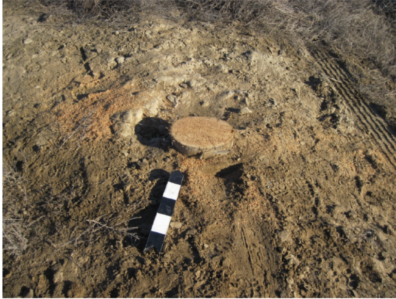
Figure 39. The poles were cut off as close to the ground as possible (azimuth north).
