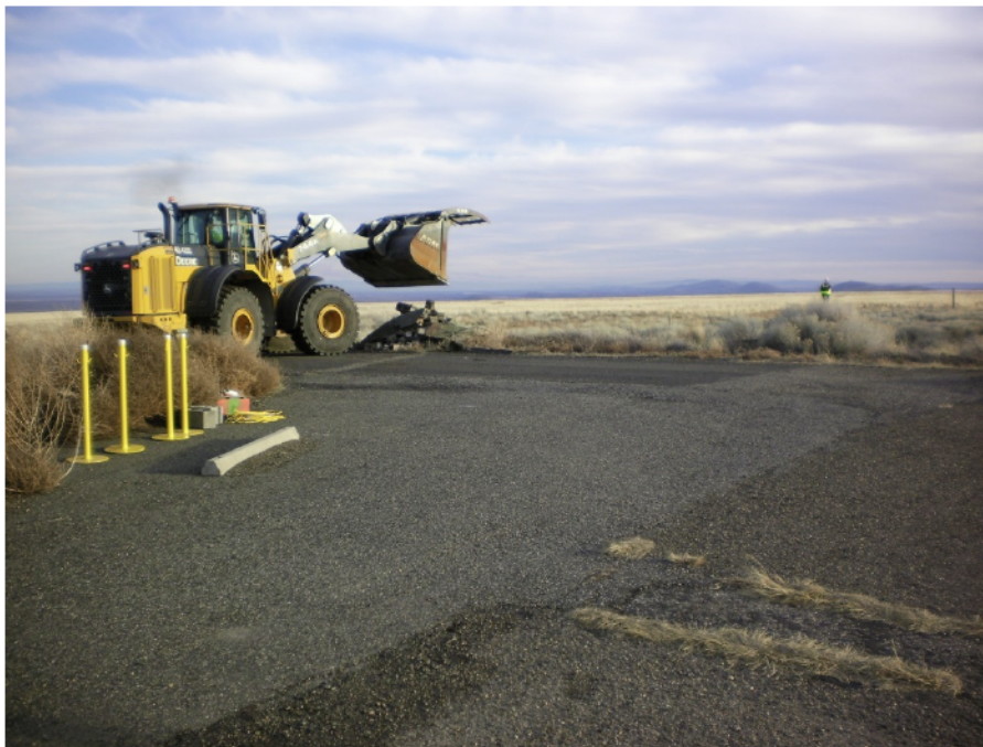
Figure 23. The guardhouse was demolished within its own footprint and loaded into a debris container (azimuth south).
