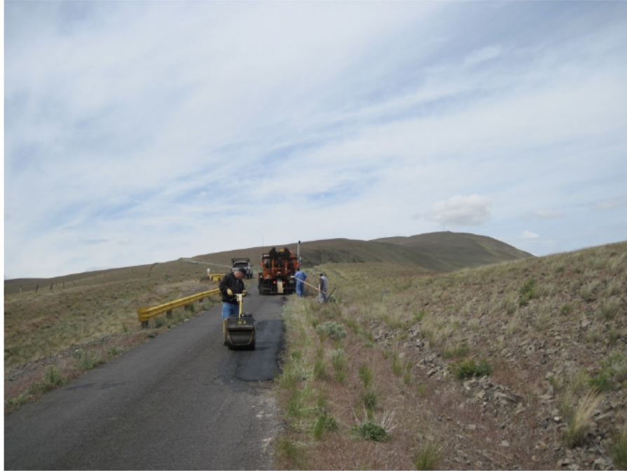
Figure 34. Crews patch and repair linear road deterioration (azimuth north).
