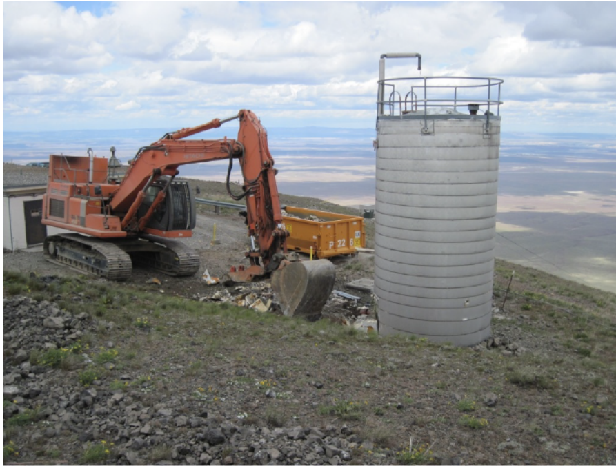
Figure 13. The small shed was demolished, and a trackhoe placed the larger pieces of debris in a dumpster (azimuth north).
