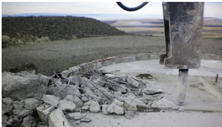
Figure 9. A trackhoe with a jackhammer attachment removed the Rattlesnake Mountain observatory foundation and slab (azimuth west).
