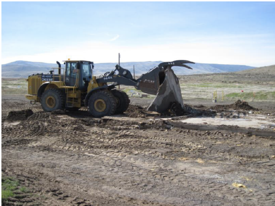
Figure 25. After demolition, the wheel loader removed the 646 Building cement foundation slab (azimuth south).
