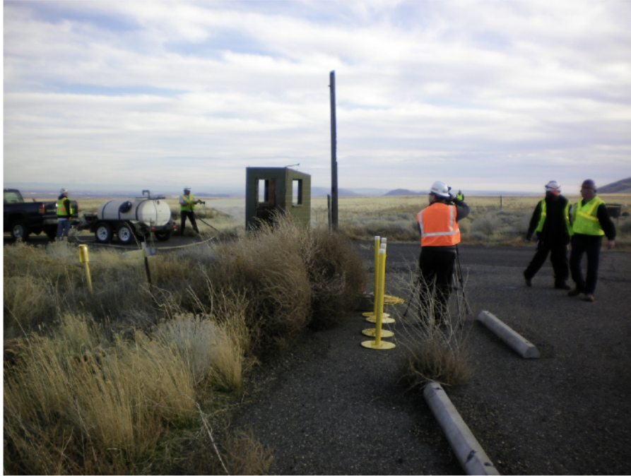
Figure 22. Crew members sprayed the guardhouse at the former Nike missile site with stabilizer prior to demolition (azimuth south).
