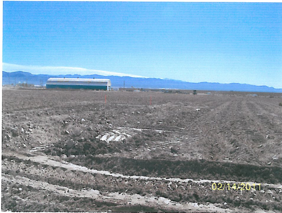
Photo 1. South Cover, ripped sub grade
