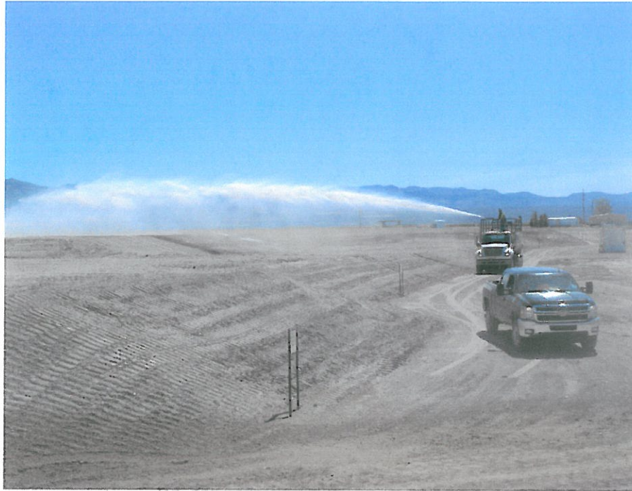
Photo 5: South Cover, truck applied soil stabilization product
