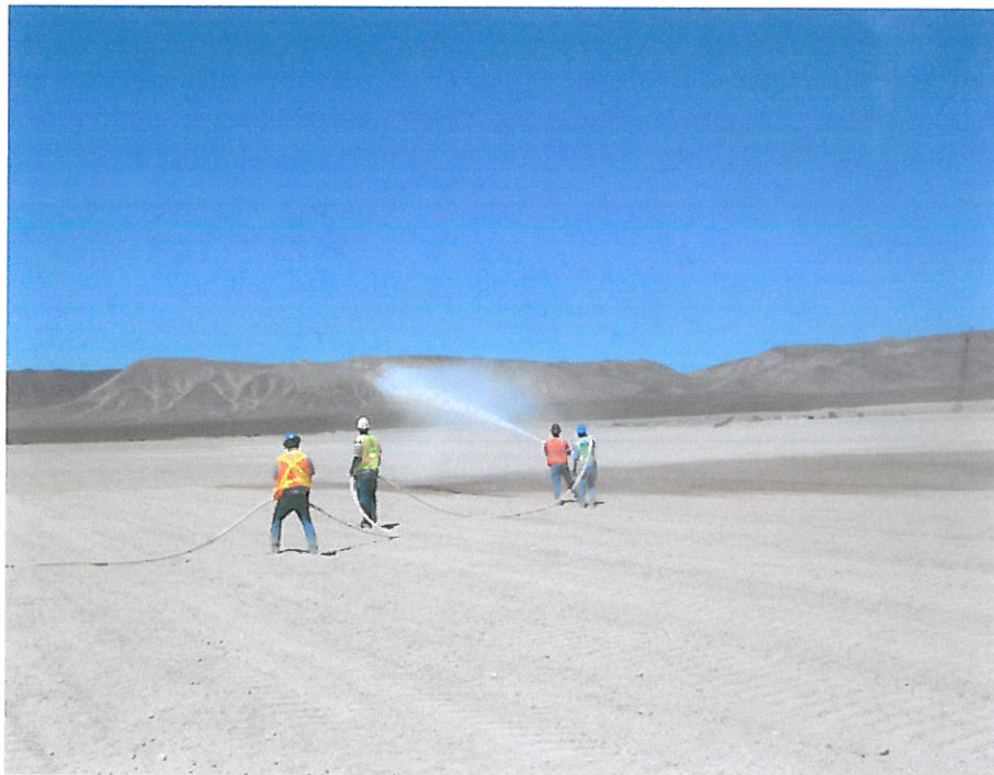
Photo 5: South Cover, truck applied soil stabilization product
