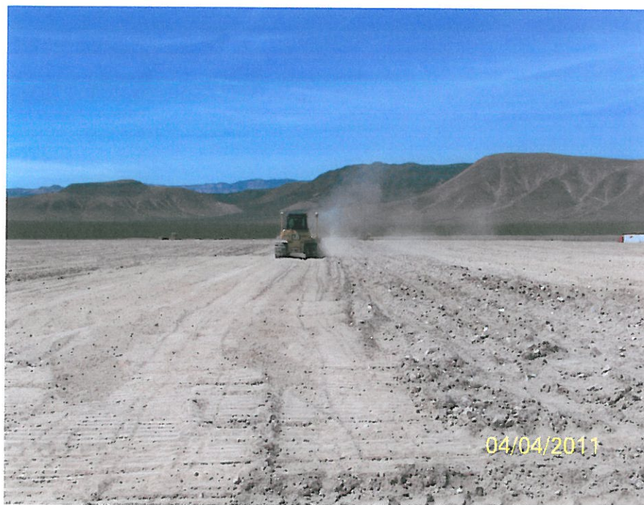
Photo 4: Track walking cover with low ground pressure D6 Dozer
