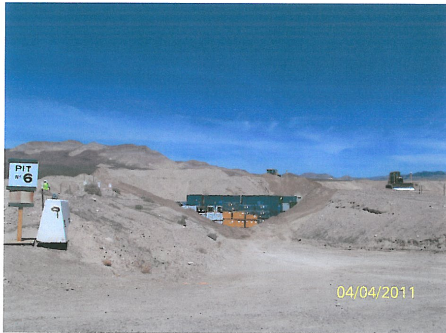
Photo 3: South Cover, Pit No. 6, Placement of cover soil
