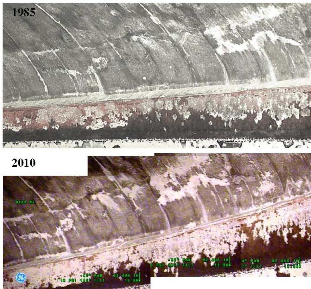
Figure 5. Comparative Photographs of Tank 241-B-102 Haunch Region
