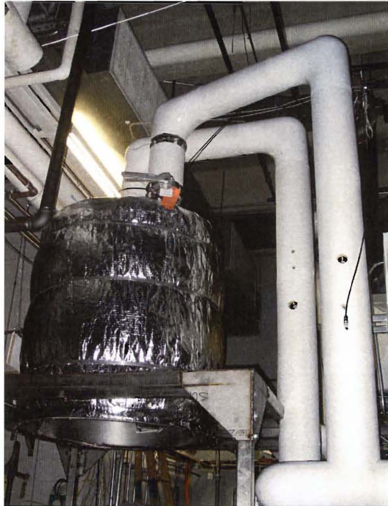
Figure 1.10. View of the installed sulfur impregnated activated carbon bed.
