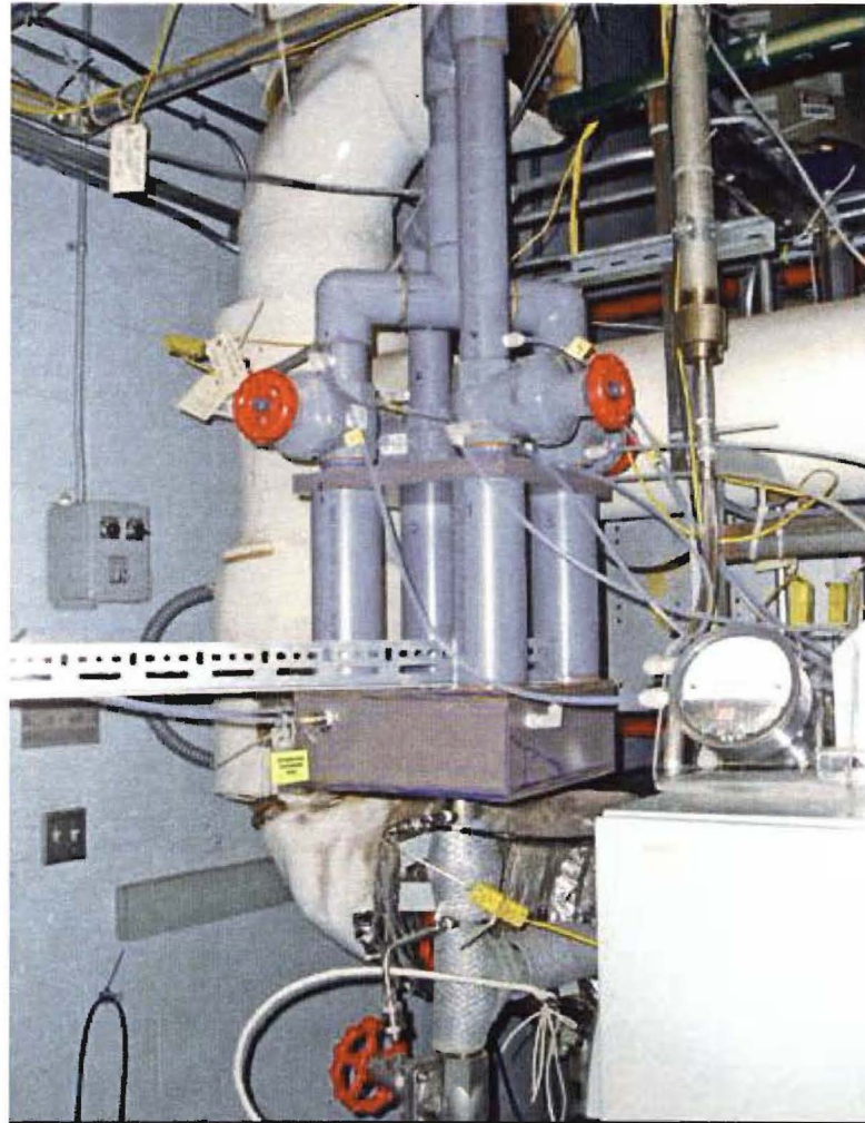
Figure 5.117. View of the filter media assembly.
